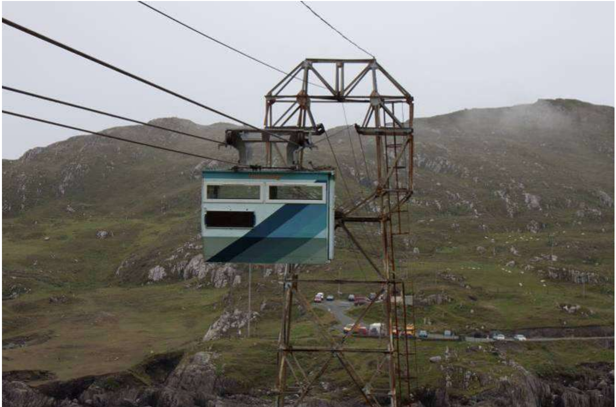
Dursey Island Cable Car, Co. Cork (antiquated and sub-standard): 400m long.
