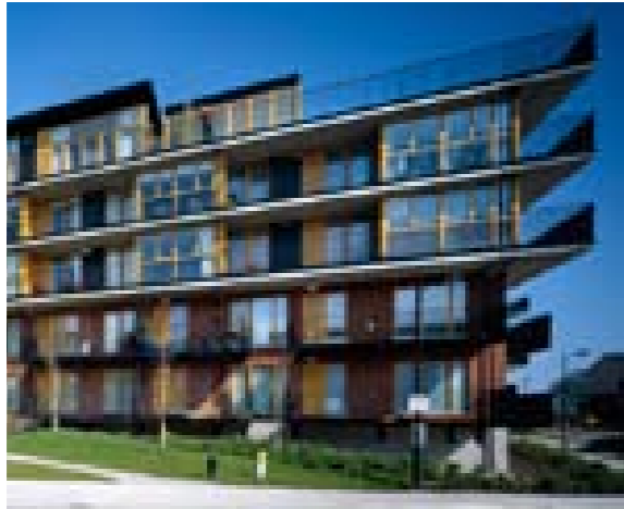
▲ Building follows the movement of the land
