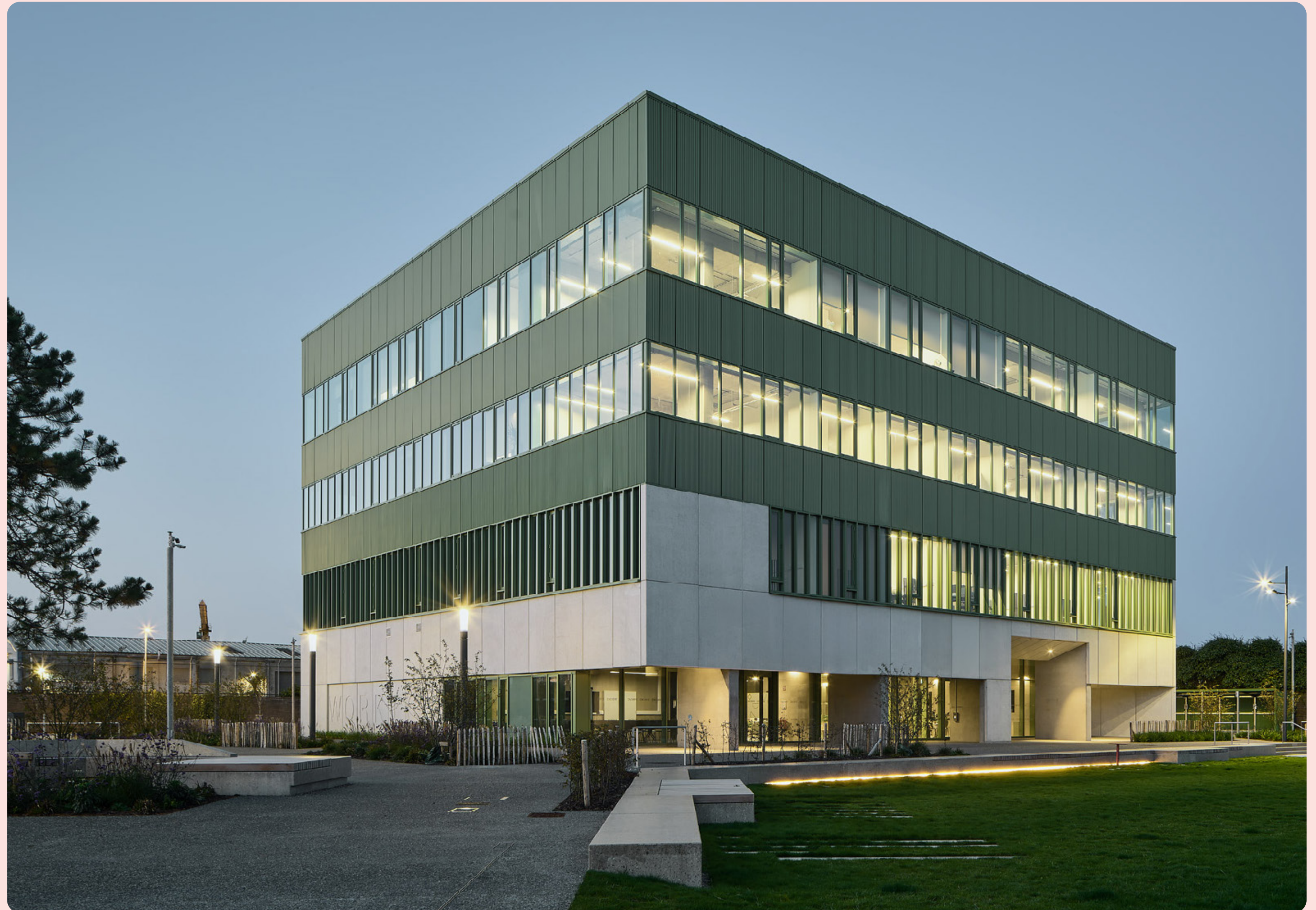
Work IQ Innovation Centre for Technology and Enterprise Growth
