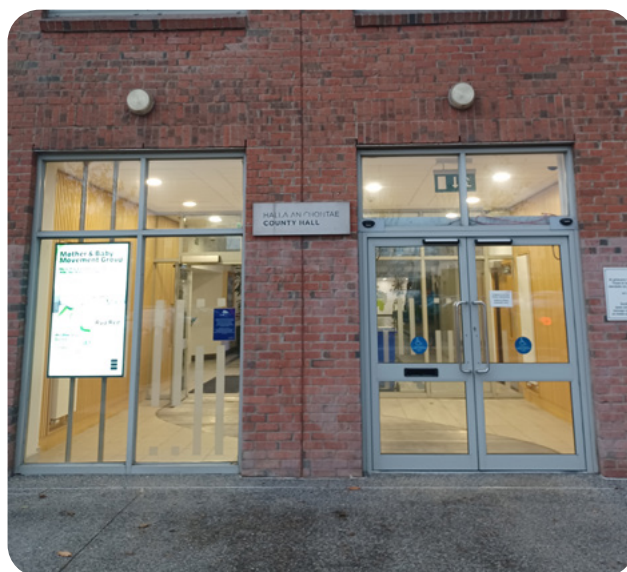
Side entrance to County Hall
