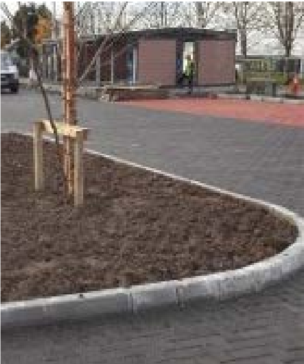
Soft landscape areas are set below kerb level at this permeable paving installation. Almac Car Park, Limerick, Ireland.
