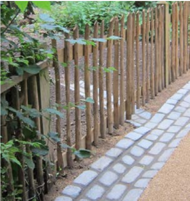
A granite sett channel collecting and conveying runoff.
