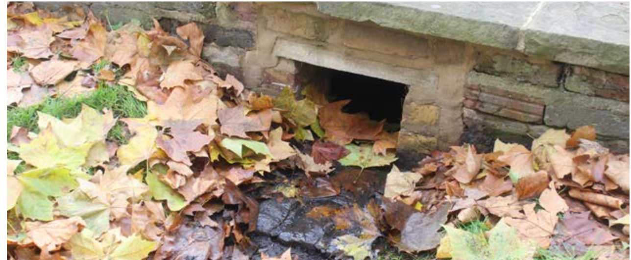
Polluted silts collecting from a busy road at an inlet apron allows for easy removal
