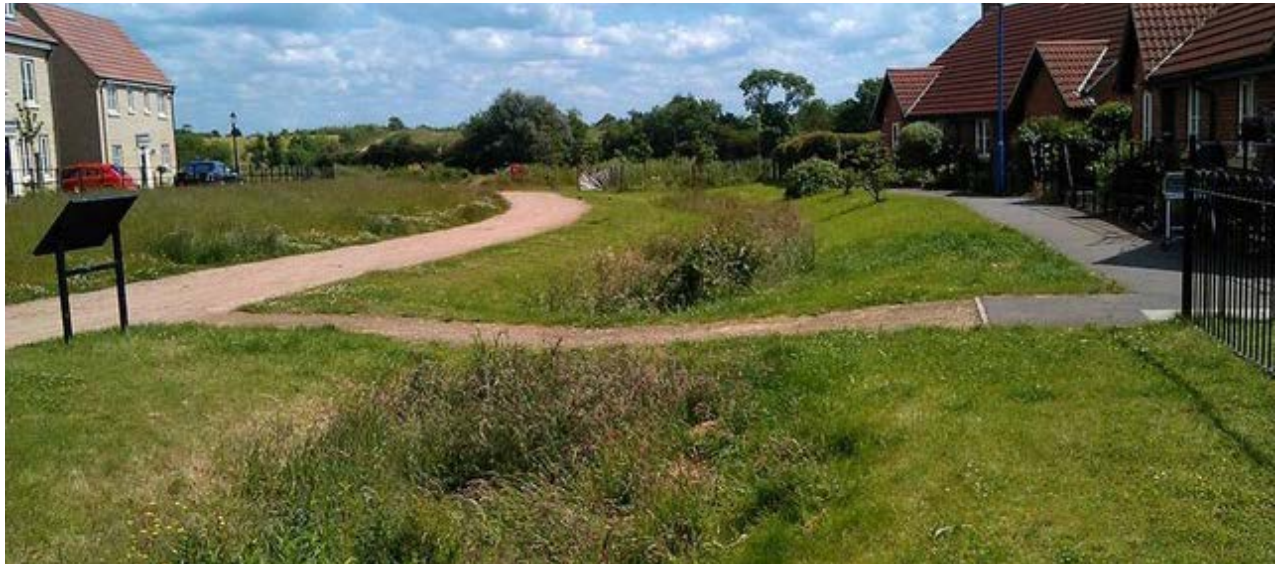
Exceedance routes are clearly visible in this housing development with dipped paths allowing exceedance flows to pass safely to the next part of the swale.
