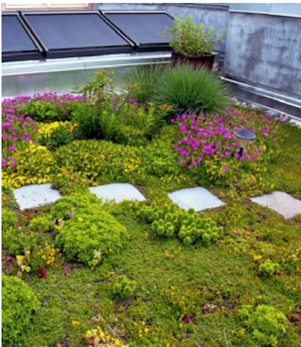
Green roofs can attenuate rainfall runoff where the outlet has a flow control ( Blue roof ).
