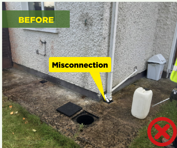
Typical domestic misconnection
