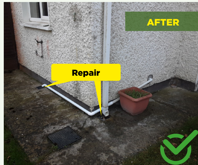
Replumbed and corrected
