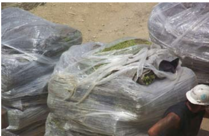
Figure 3.1 Pallets of Sedum matting ready to be rolled out (Courtesy C Sosman)
