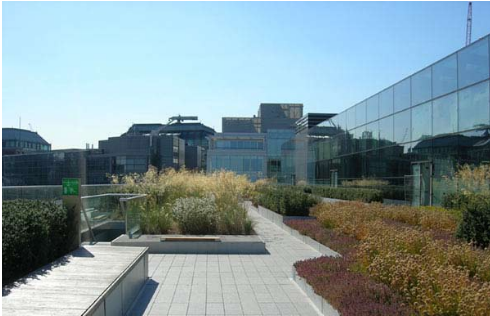
Figure 4.1 Semi Intensive Green Roof in London
