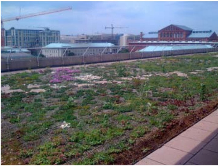
Figure 1.5 Extensive Green Roof in Washington (courtesy C Clark)
