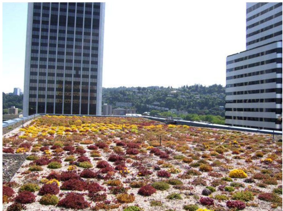
Figure 4.6 Close up on Portland Council building green roof
