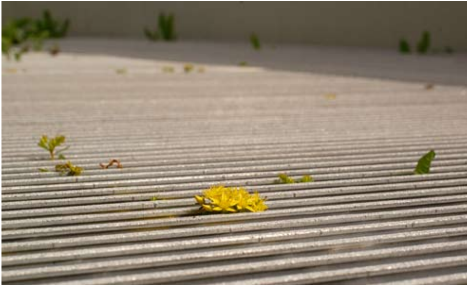
Figure 2.13 Side view of the walkway grill with Sedum plants growing through (Courtesy D Saunders)
