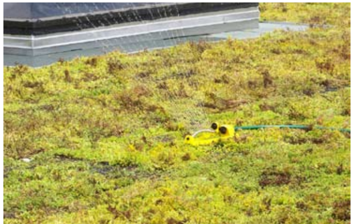
Figure 3.3 Irrigating the Sedum matting (Courtesy C Sosman)
