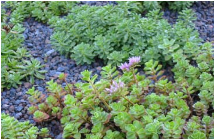
Figure 3.5 Sedum plants on an extensive green roof (Courtesy C Clark)
