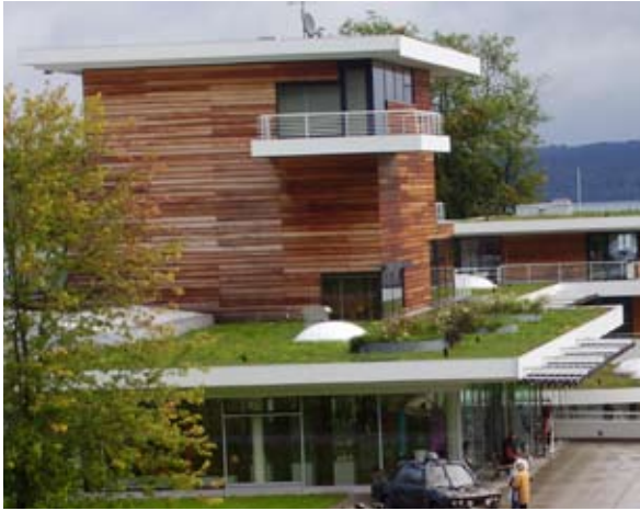
Figure 2.8 Extensive green roof on several levels in Munich, Germany
