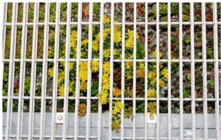
Figure 2.12 Sedum plants placed underneath the walkway grill on the ASLA green roof (Courtesy D Saunders)
