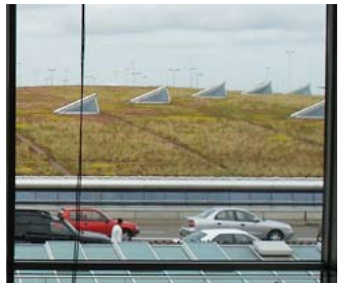
Figure 1.1: Carpark cover, Schiphol Airport, Amsterdam (© Erik van Lennep)
