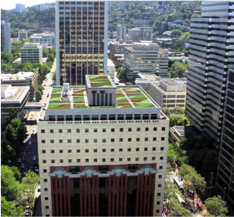
Figure 4.5 Green Roof on City of Portland, Bureau of General Services
