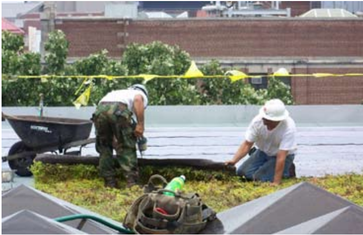
Figure 3.2 Sedum matting being applied to roof (Courtesy C Sosman)
