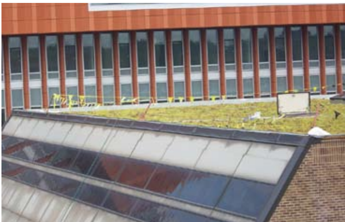
Figure 3.4 The completed extensive Sedum green roof (Courtesy C Sosman)
