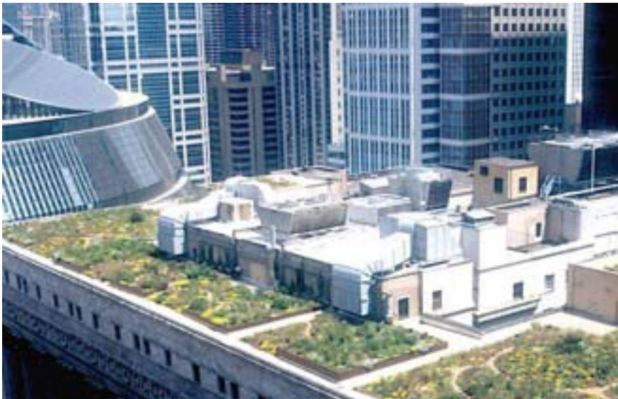
Figure 4.4 Simple Intensive Green Roof on Chicago City Hall
