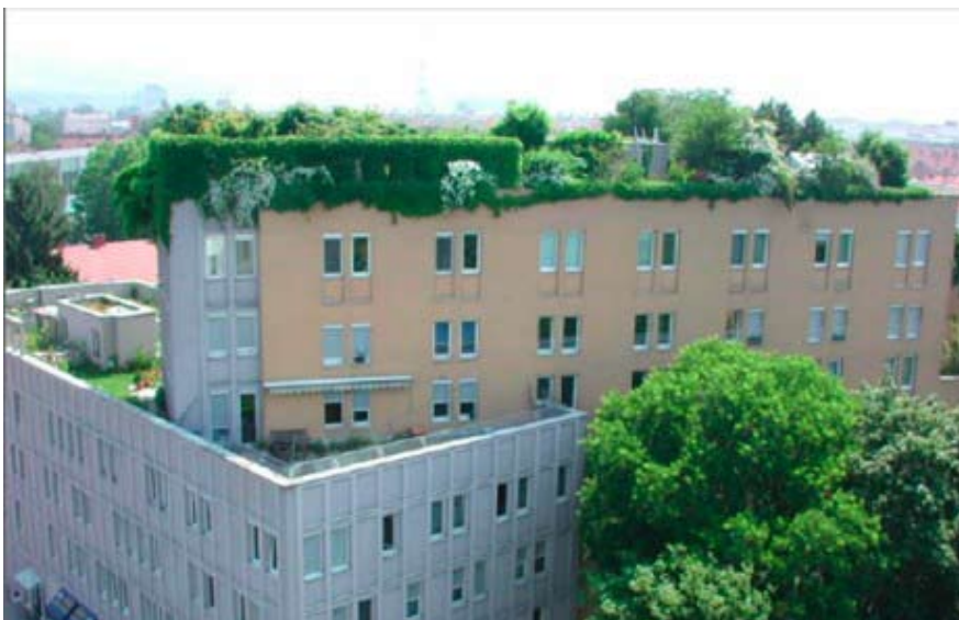
Figure 4.3 Example of green roof on an apartment complex in Linz
