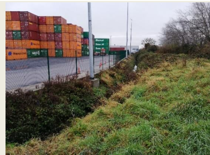
1) Looking DS: Industrial land use to the north; the Grand Canal is to the south. Channel is over-deepened and embanked.
