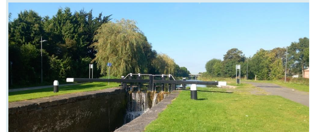
The Grand Canal environment at Ninth Lock Road
