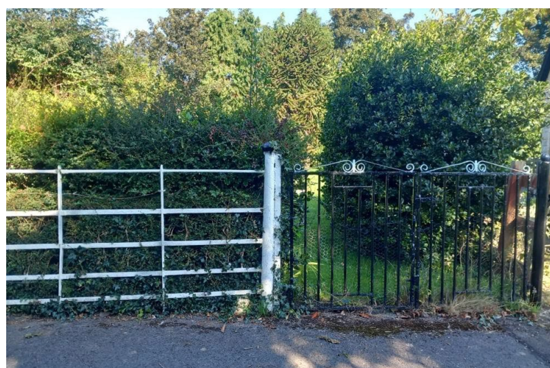
Plate 2 Front Garden boundary walls feature original wrought iron railings.
