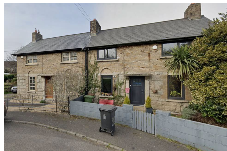
Plate 3 Incremental alterations, such as changes to fenestration design and loss of front boundary walls have a major impact on the character of the historic streetscape.
