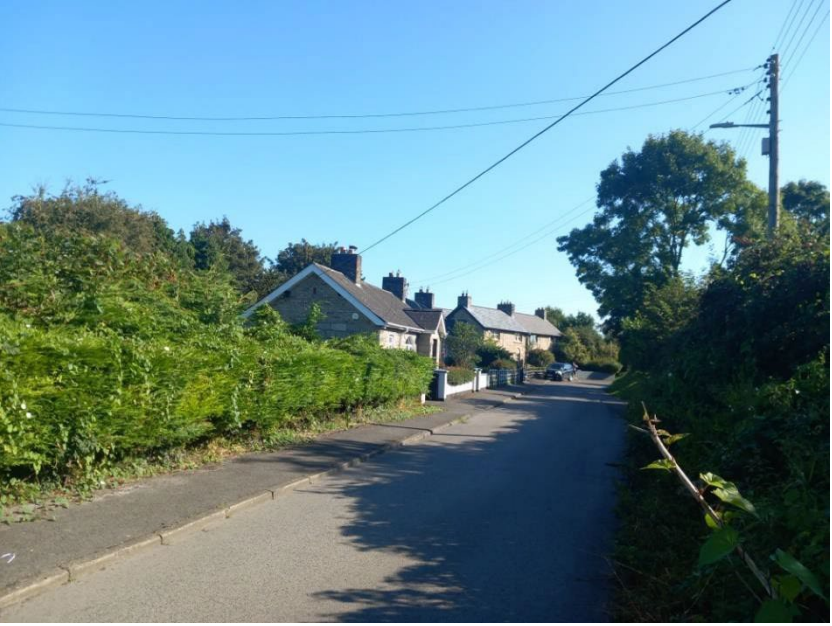
Plate 5 Informal planted boundaries contribute to the rural character of the lane. The overhead wires and cables attached to chimneystacks detract from the visual amenity of the streetscape.
