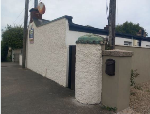
Cylindrical pier of the former 18 th century farm grouping on New Road
