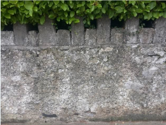
Limestone wall on east side of Tower Road. Roughcast render on limestone, with distinctive cock and hen coping
