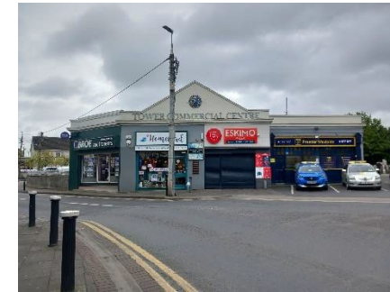
Tower Cinema, a culturally significant structure of early 20 th century origin
