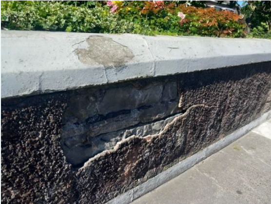
Early 20 th century intervention, at the southern end of Tower Road and similar along the northern side of Monastery Road, with chamfered coping (now painted) and pebbledash render applied to the earlier limestone wall
