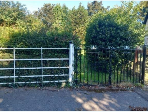
Simple vernacular wrought iron gates and railing positively contribute to the public realm
