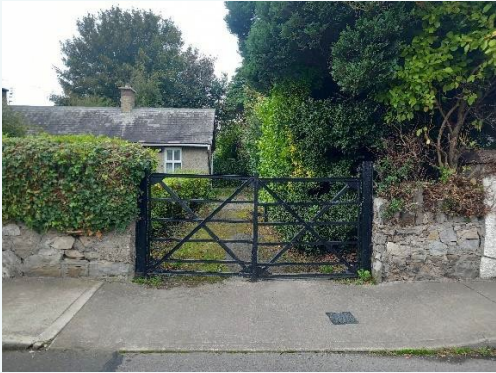
Rubble limestone walls with traditional wrought iron gates
