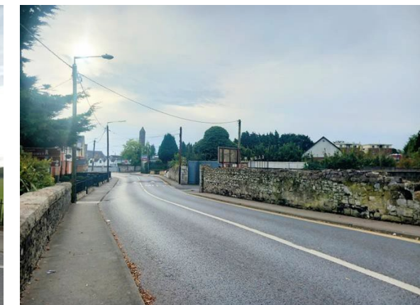
View 6 On approach from Old Nangor Road
