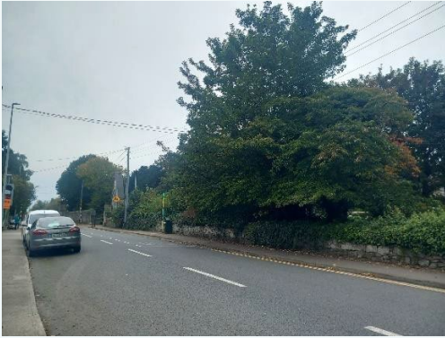
Rubble limestone wall determining character of street
