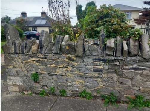
Fieldstone copings in rubble limestone wall
