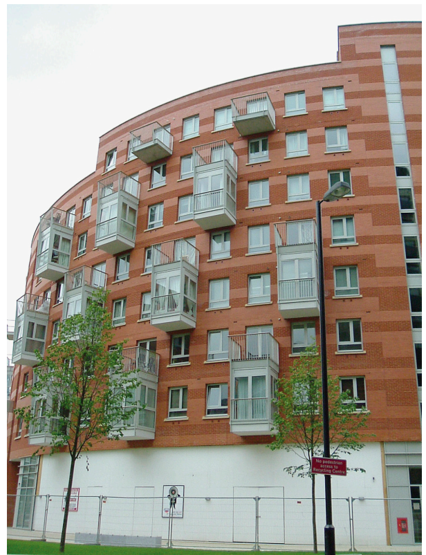
Figure 13: This North London development (architects CZWG) has staggered balconies to minimise obstruction to living rooms. Where a balcony is above a living room the obstructed area has been modified to form an unobstructed bay window.
