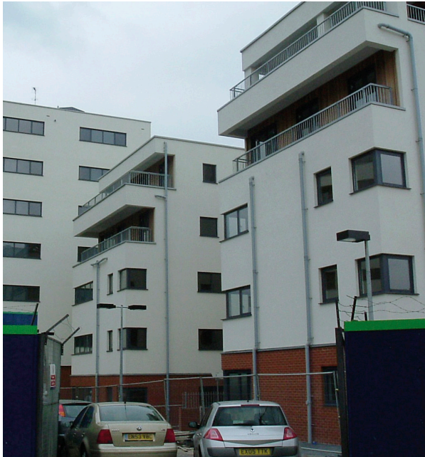
Figure 8: A white finish to external walls, as in this North London development (architects Sheppard Robson), can increase reflected light. However, windows will tend to reduce the overall effective reflectance.
