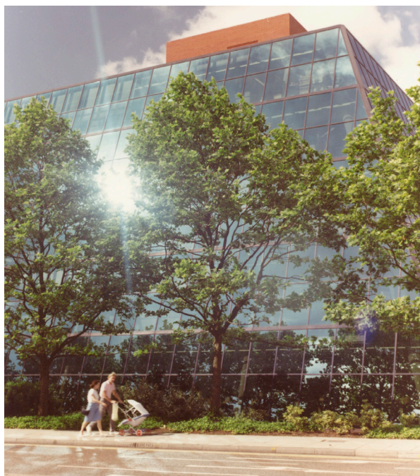
Figure 41: Solar dazzle reflected from a glazed façade
