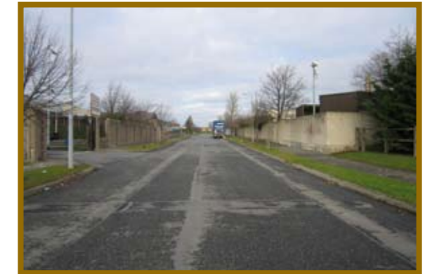
Industrial units within Whitestown Industrial Estate looking south along Whitestown Drive.
