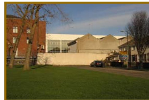
Flank wall at the end of a cul-de-sac.
