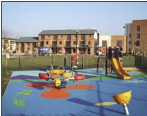
Toddler's play area within the Public Park currently under construction
