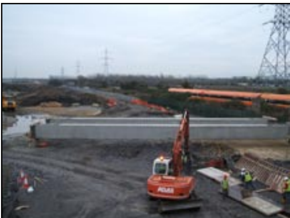
View eastward along route of A.L.R. adjacent to Dublin/Kildare railway line
