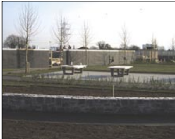
Outdoor table tennis area within the Public Park currently under construction
