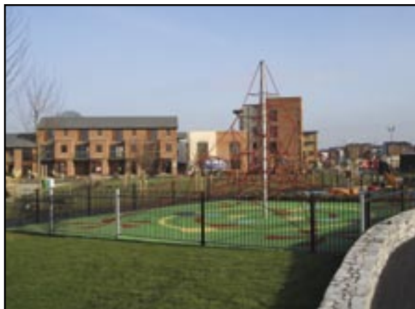
Children's climbing web within the Public Park currently under construction
