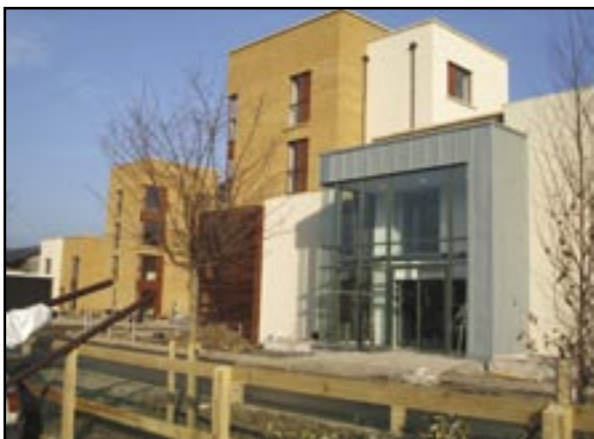
Marketing Suite / Information Centre currently under construction within Adamstown Castle
