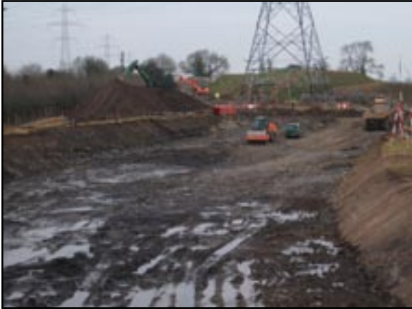
View westward along route of A.L.R. towards Adamstown Castle
