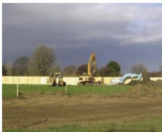
Boundary fencing between the site and Finnstown House Hotel
