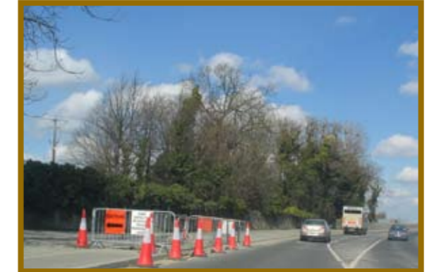
ITT side of Greenhills Road looking north.
