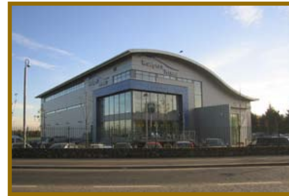
Gymnasium fronting Greenhills Road.
