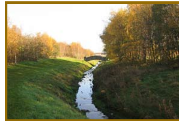
Pedestrian bridge over the Tymon River within Bancroft Park.
