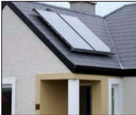
Example of solar panels on an extension.
