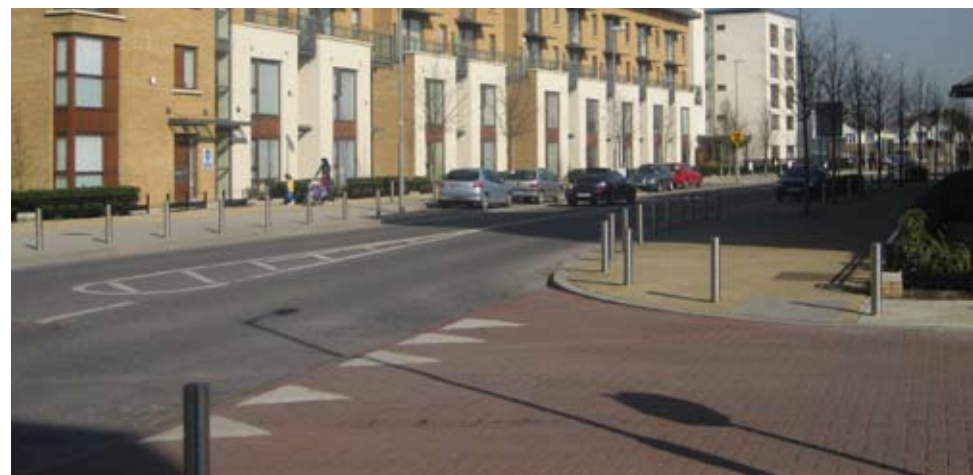
Example of a raised entrance treatment to slow traffic entering a 30 kph Side Street from a 50 kph Avenue.
