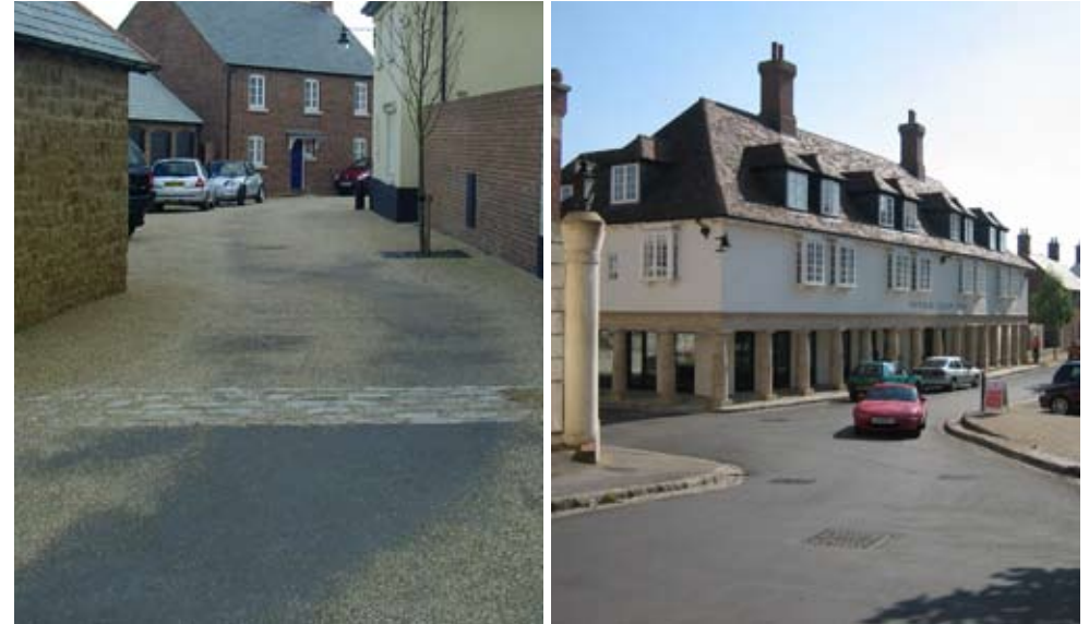
The shared street philosophy of Poundbury with its limited sightlines, narrow winding carriageways, shared surfaces and frequent junctions was considered radical at the time of its conception and have proved a great success.
