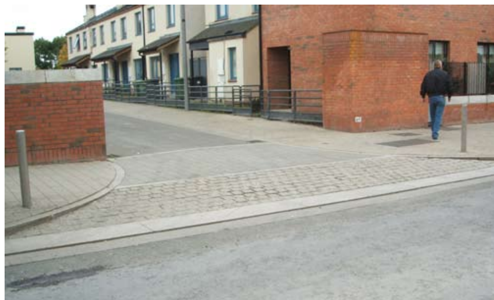
Example of entry treatment designed to slow drivers and maintain a sense of pedestrian priority.
