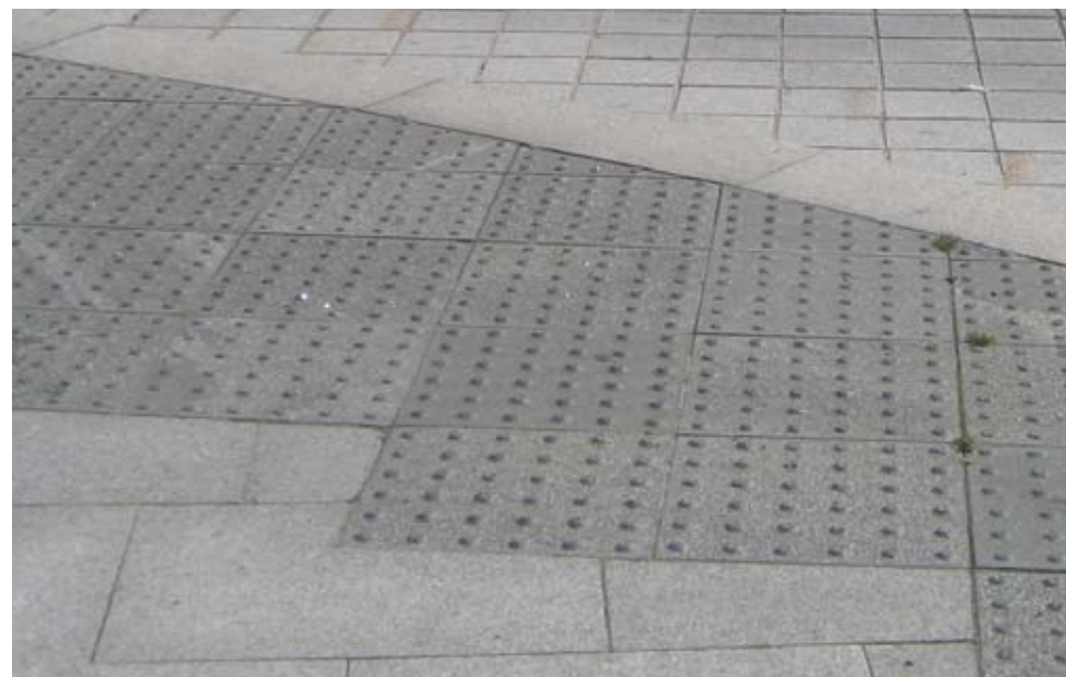
An example of grey blister paving used at a signalised crossing in a high amenity area.
