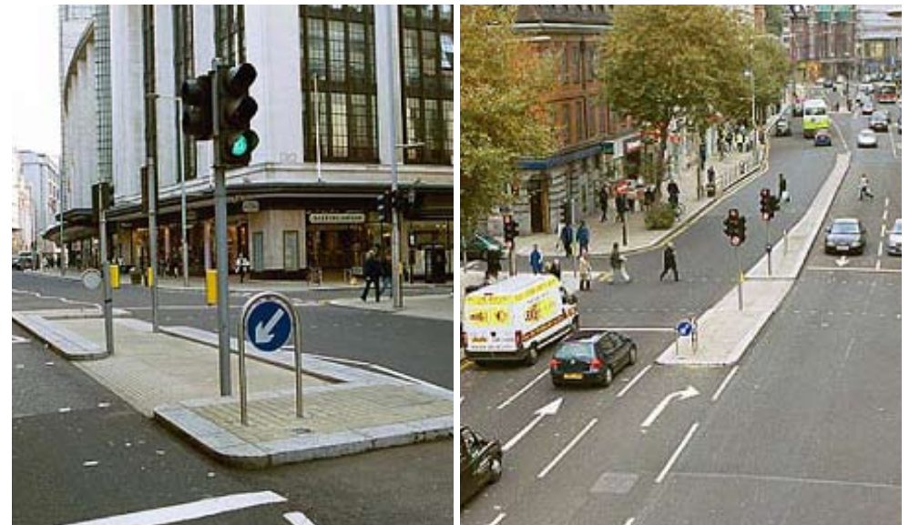
The improvements to Kensington High Street which include the removal of guard railings and excessive signage, along with paving and lighting upgrades, has modified driver behaviour and reduced accident rates (Image source www.rbkc.gov.uk ).
