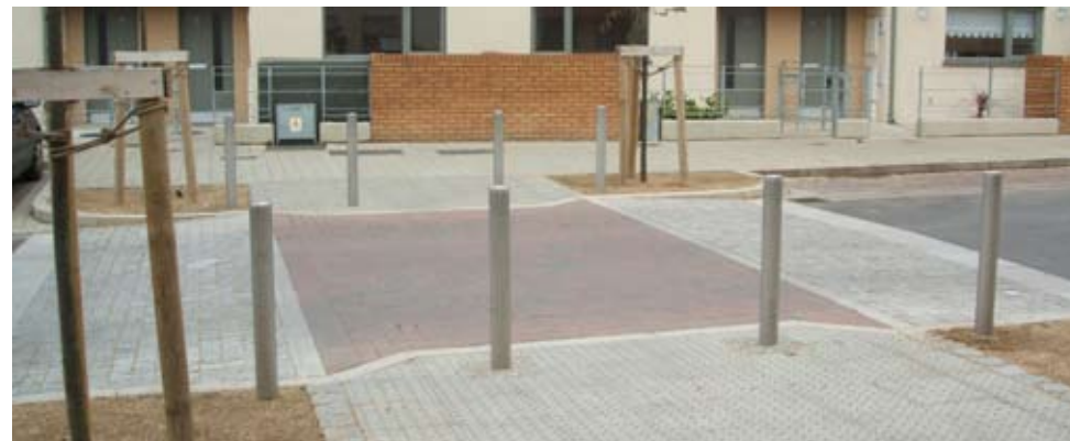
An example of a mid block pitch point with a surface change and vertical deflection which also functions as an informal crossing.
