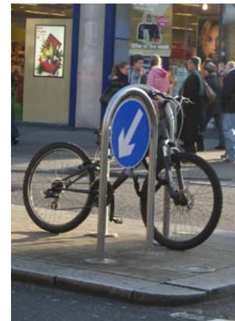
Examples of the use of hoop bollard that can be used to direct traffic and provide a sense of protection for pedestrians.
