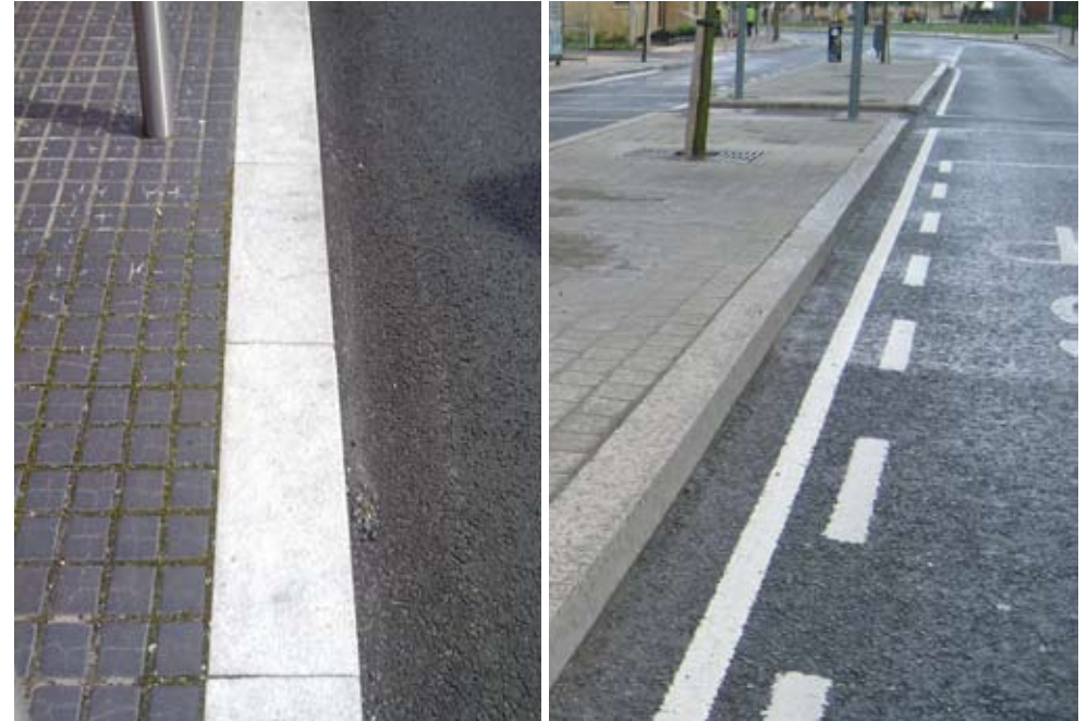
Examples of distinctive kerb elements. The example to the left is constructed of reconstituted stone within a higher specification area. The example to the right is constructed with concrete blocks along an Avenue within Adamstown.
