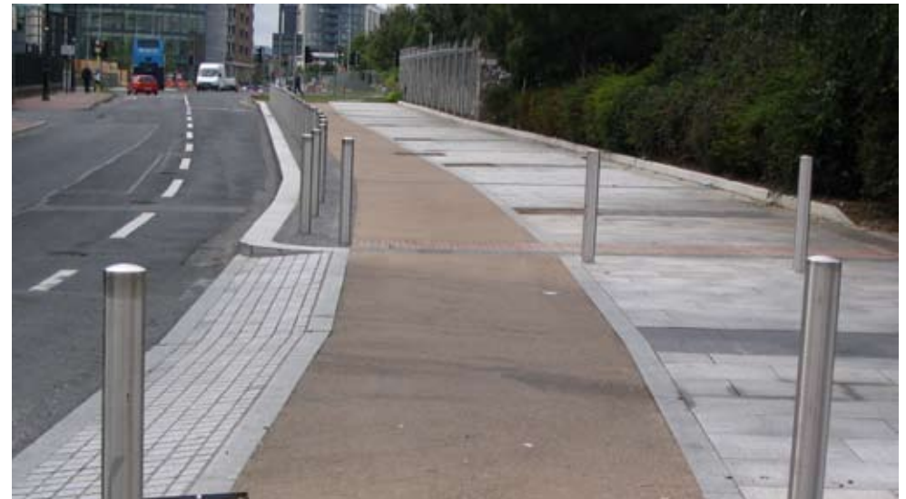
Example of a dished kerb where kerb lines and footpath levels are maintained.
