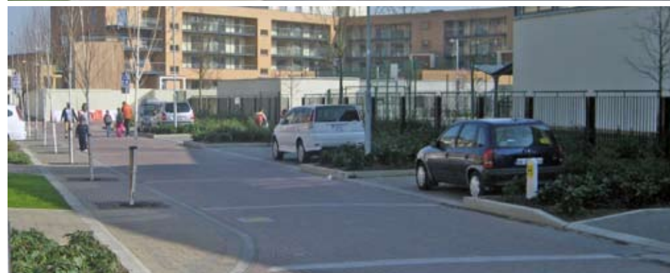
Images of the different carriageway designs within Adamstown. From top 50kph Avenue; 30 kph Side/Back Street and 10 kph Homezone.
