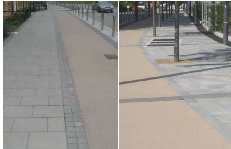
Smooth cut block paving pedestrian paths (left: concrete, right: reconstituted stone) and cycle path finished in an asphalt buff. The example to the left is a high specification finish along an Avenue within Adamstown. The example to the right uses the higher specifications along a strategic pedestrian/cyclist link within a town centre.
