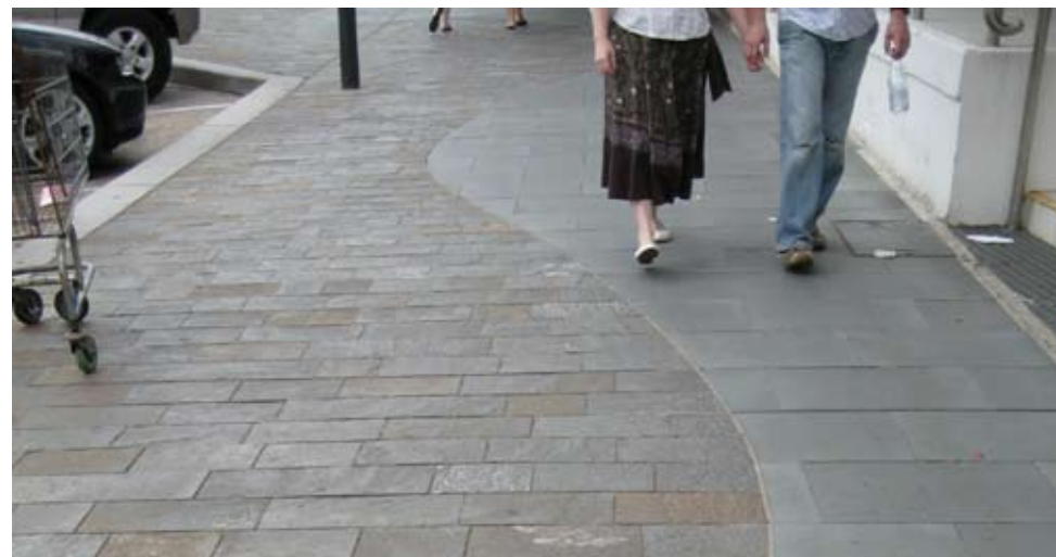
Wide decorative stone block paving within a highest specification environment (district centre) to cater for higher pedestrian volumes and emphasise the areas civic importance.
