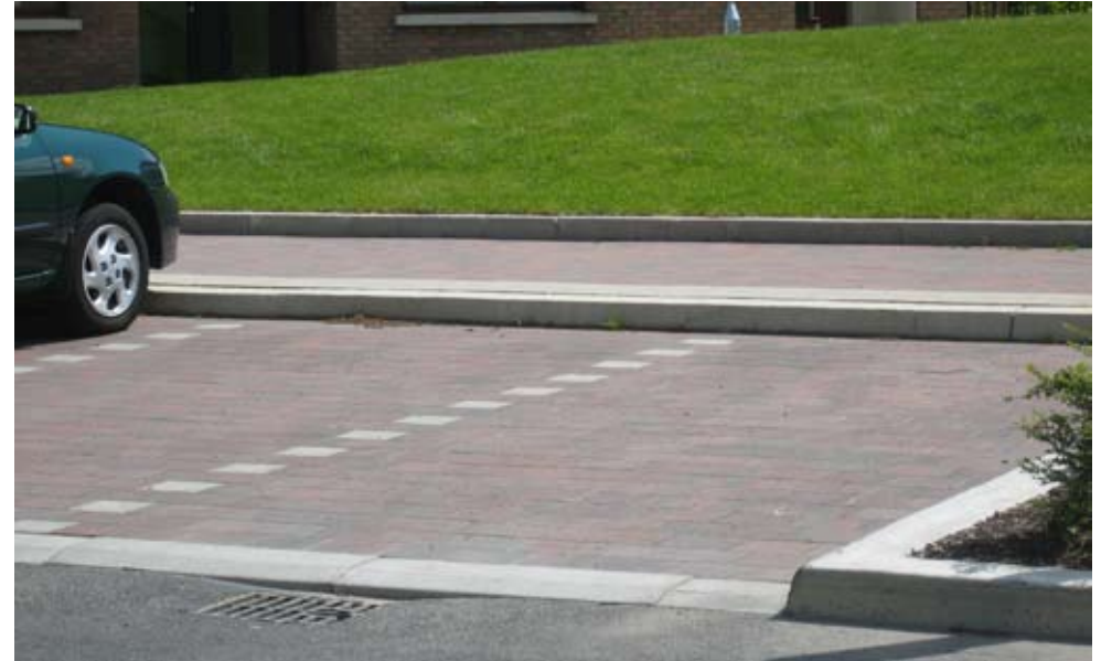
Example of on-street parking bays within Adamstown finished with block paving. Contrasting paving is used to demarcate the parking area as a whole and/or individual parking bays.
