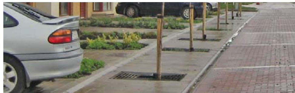
Verge adjacent to shared zone which provides an area of pedestrian refuge, allows for vehicle overhangs and facilitates the planting of street trees.
