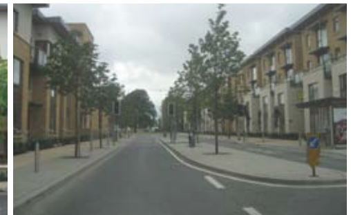
Continuous Street Wall
