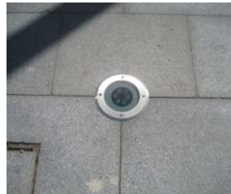
An example of a small spot light provided within the path of a higher specification amenity area.
