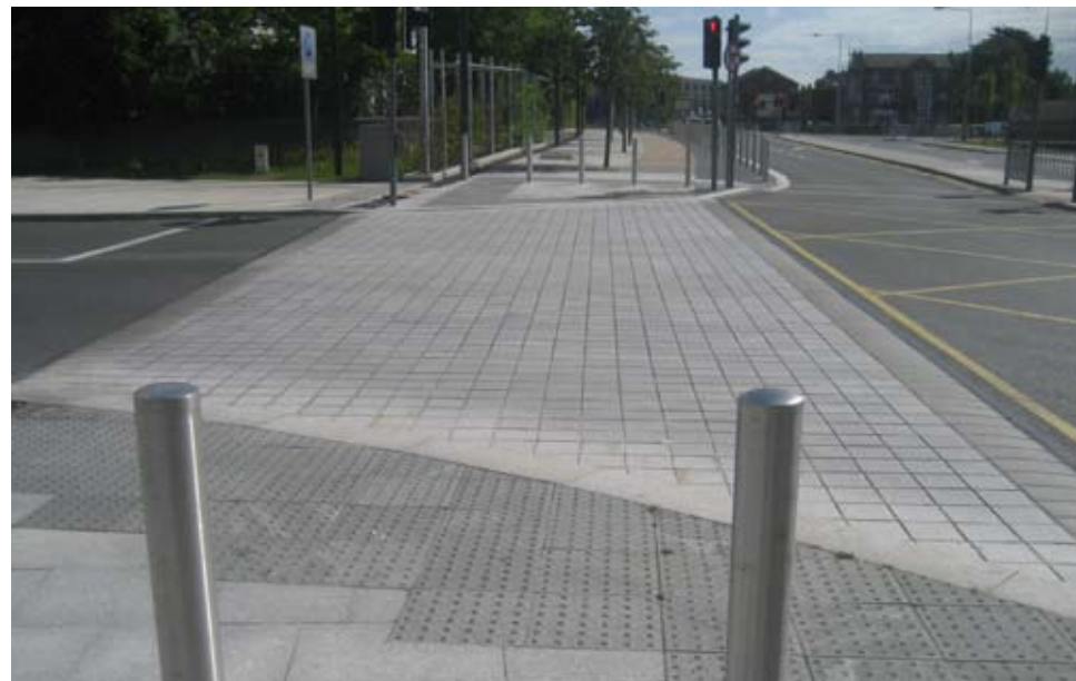
Example of a pedestrian crossing where paving has been continued across the carriageway to alert drivers and maintain a sense of pedestrian priority.
