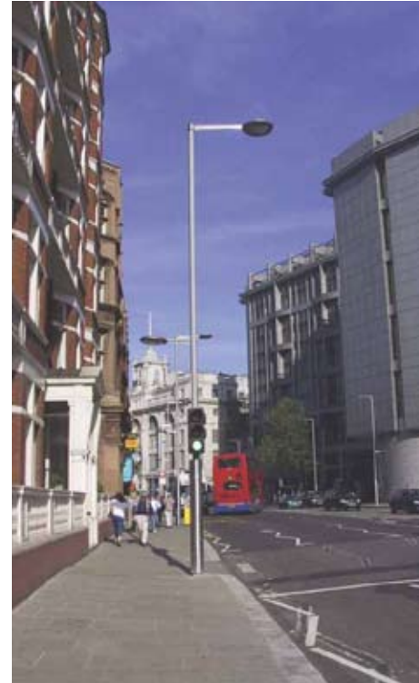
An example of a dual light with a lower lamp over the pedestrian footway. Source: http://www.rbkc.gov.uk
