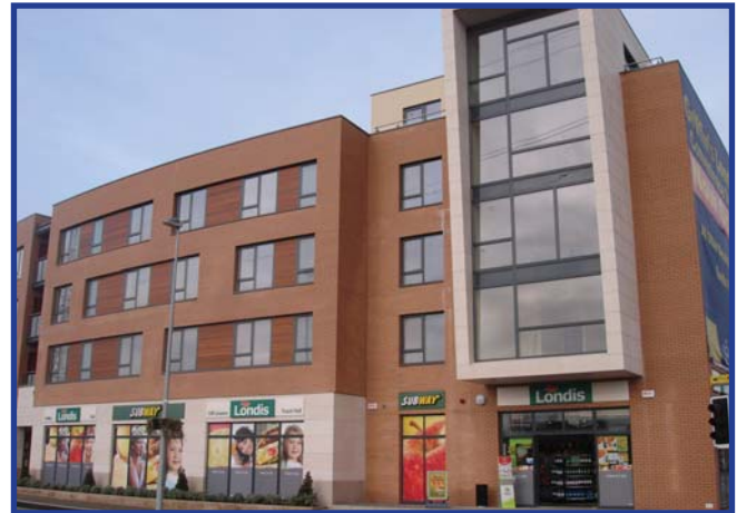
Photo of Sentinel Building containing Londis convenience store
