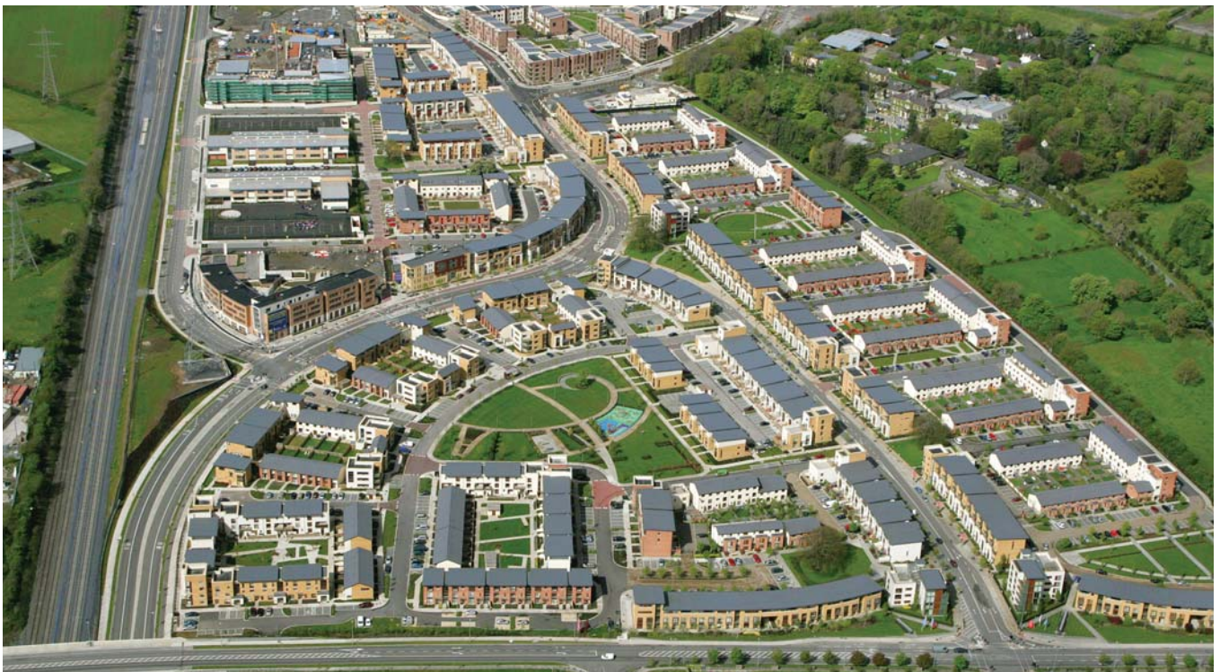
Aerial photo courtesy of Castlethorn Construction
