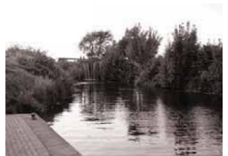
The Grand Canal 9th Lock gate
