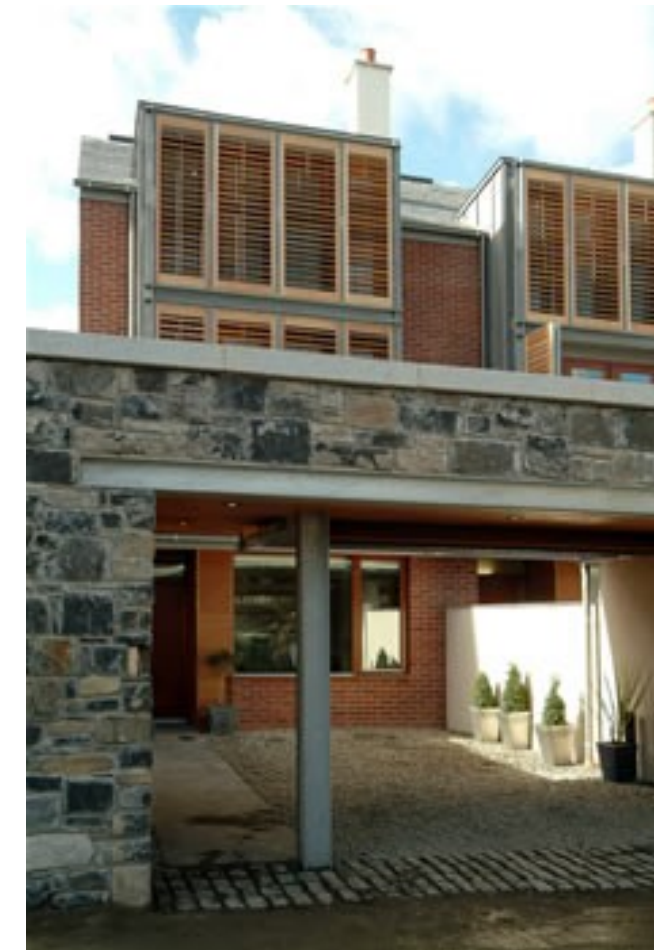
Fig 4.2: An example of the use of privacy screens at first and second level.
