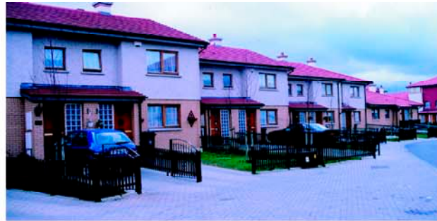
Figure 5.13. Housing with Shared Surface Access, Brookfield
