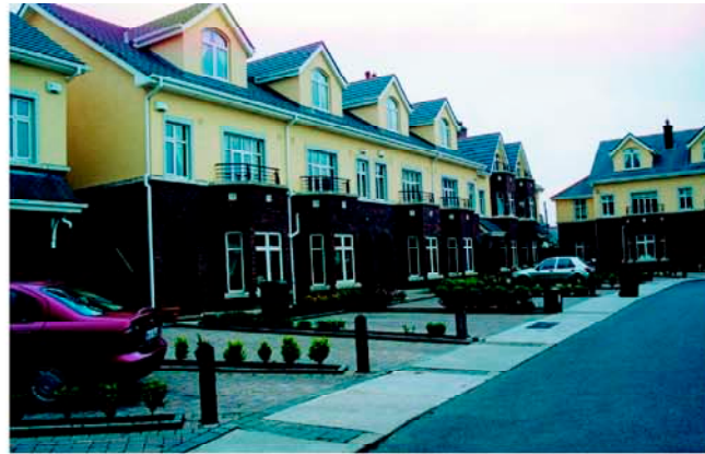
Figure 6.18. Private Car Parking Bays
