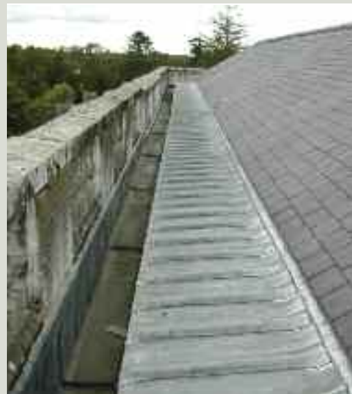
Welts to lead flashing to the vertical face of the parapet wall. Note the steps in the lead gutter and the rolls in the lead apron on the lower portion of the roof slope
