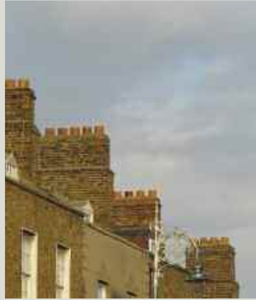
The typical Georgian streetscape of the late-eighteenth century is characterised by the suppression of the roof as an architectural element. Roof pitches were reduced to a minimum and architectural devices such as double roofs and parapet walls were used to ensure that the roof stayed out of sight from street level
