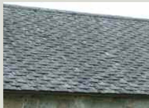
A method of slating sometimes referred to as 'open slating', 'hit-and-miss slating' or 'Scottish cant'. This slating pattern economised on the number of slates used and was primarily used for outbuildings. It is difficult to repair without face-fixing and the amount of exposure of slate surface can make the slates brittle for reuse
