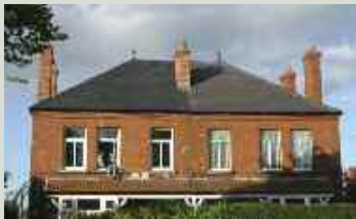
A recently replaced Welsh slate roof (to the left) adjoining a historic one (right), where the difference of character, colour and texture can easily be seen
