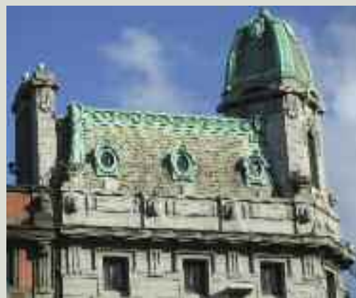
Copper used for the decorative trimming of architectural details on a mansard roof and dome, its green hue complementing the pale grey of the slate and stonework
