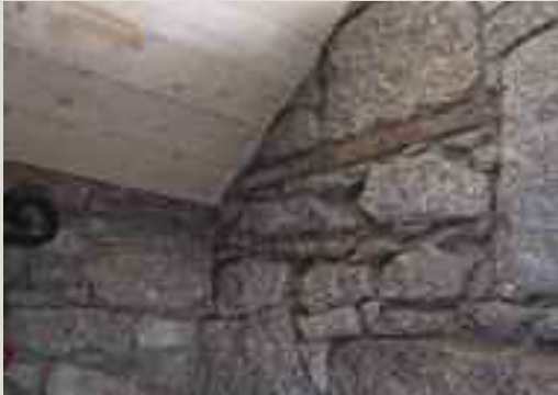
Halved wall plate plus timber strap bedded into a cross wall
