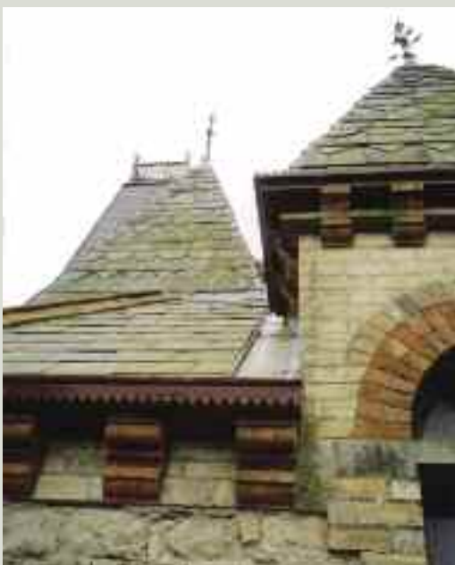
Decorative finials and ridge tiles were added for decorative effect and contrast. However, sometimes the use was also functional, for example when concealing a vent to the roof space
