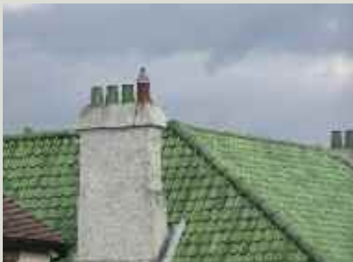
Glazed terracotta chimney pots are unusual, but examples with green, black and dark brown glazes can still be found with a simple roll-top detail. In this example, the bright green glazed pots match the glazed roof tiles. Further variations included tall dark brown terracotta pots with serrated tops and short plain black pots like crowns
