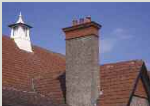
An Arts and Crafts style clay-tiled roof with tile hanging to the upper part of the gable
