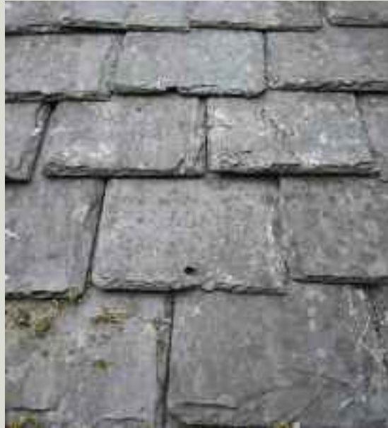
Slates are swung back into place after works
