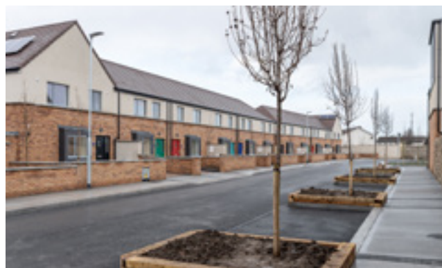
Construction of 238 new homes
