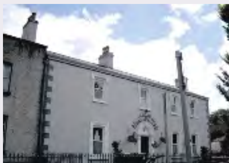
Muintir Na Tire, Lucan was grant aided for roof repairs
