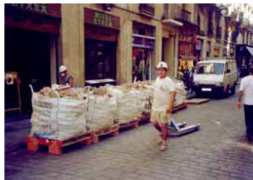
Source separation of recyclable C&D waste
