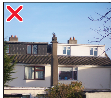
Avoid creating the impression of a 'flat roof' with badly designed roof extensions
