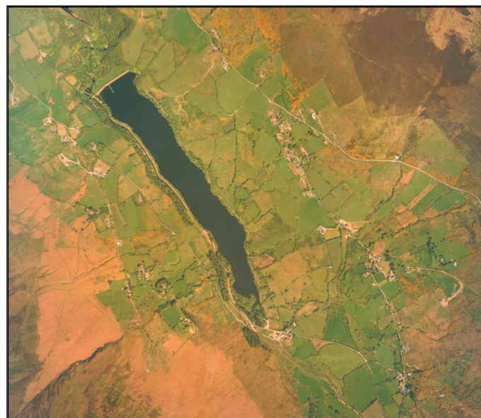
Aerial view of Upper Bohernabreena Reservoir
