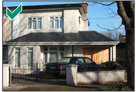
A front extension that complements the distinctive style of the original house. Note how the garage door has vertical boarding and is sufficiently recessed behind the front wall of the extension to minimise its visual impact
