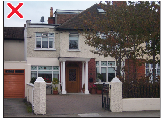
The jarring visual effect of a group of extensions to the side, roof and front of a house that do not complement original house or each other
