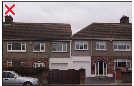
Avoid extending a hipped roof to create a gabled end over a side extension or creating a terraced effect and difficult joins between rooflines
