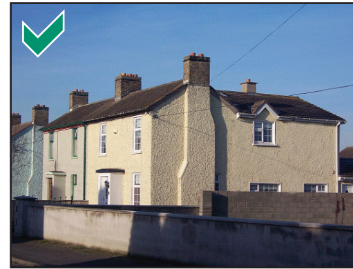
Careful attention to scale and detail is particularly important where large rear extensions are visible from public view
