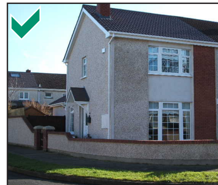
A good example of 'turning the corner'; a side extension on a corner plot that avoids creating blank elevations
