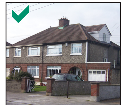
Extensions to hipped roofs should sit below the ridgelines and match or complement the materials of the main house
