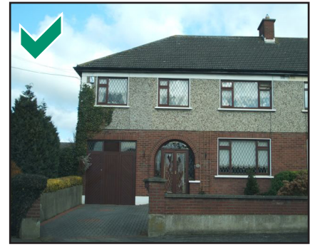
Seamless extension where materials and hipped roof match the original house
