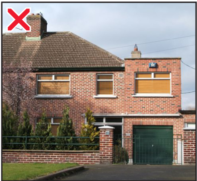
Prominent flat-roofed two storey extensions are not normally acceptable
