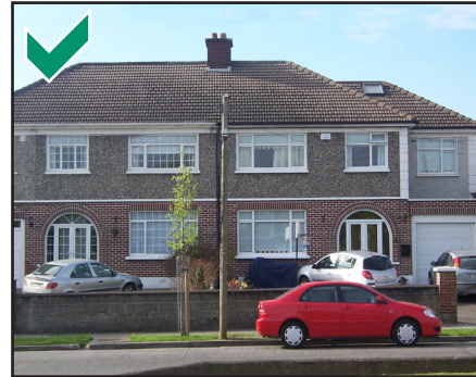
Examples of an 'ancillary' extension that reflects the hipped shape of the original roof
