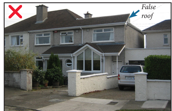
The use of a 'false' roof to the front of an extension is rarely successful
