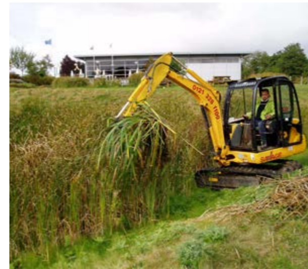
A light tracked excavator removes aquatic vegetation to de-water next to the wetland, before moving to a wildlife pile.
