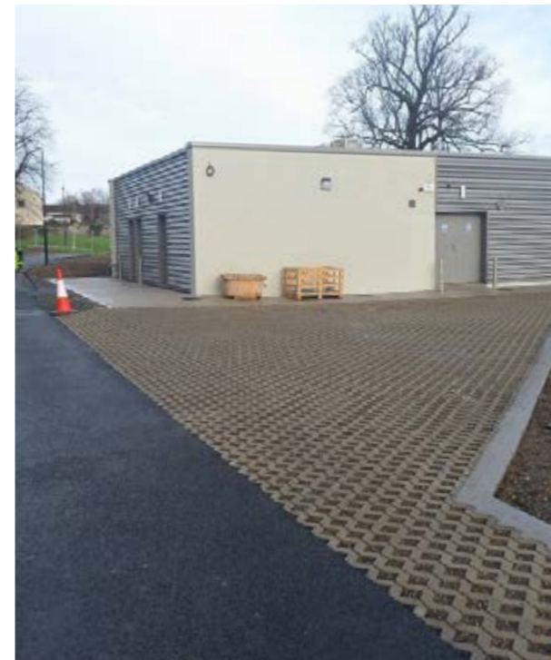
Reinforced grass paving area Dodder Valley Park Sports Pavilion (credit AOCA)
