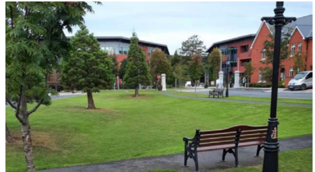
Detention Basin in public open space - The Way, Citywest Avenue
