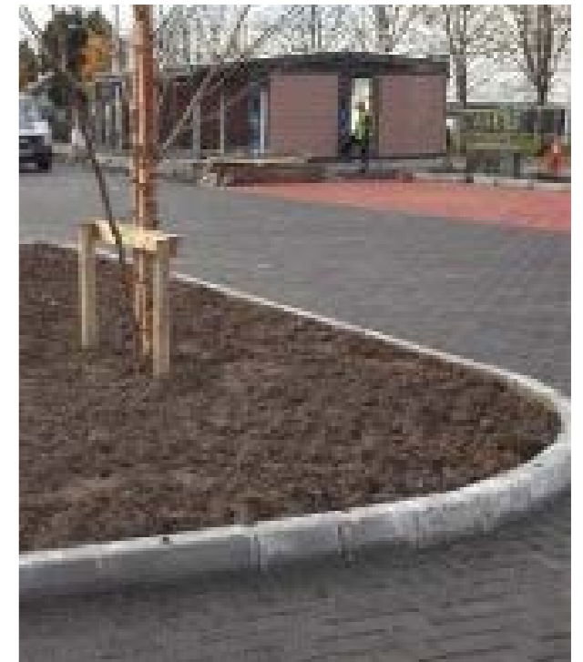
Soft landscape areas are set below kerb level at this permeable paving installation. Almac Car Park, Limerick, Ireland.
