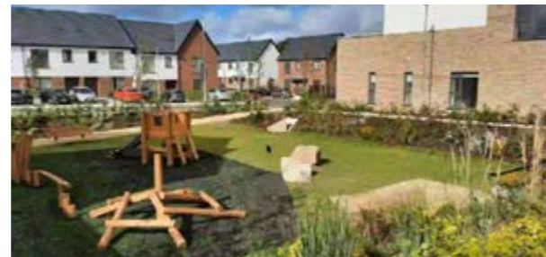
This play area provides site containment of flow which exceeds the capacity of the SuDS attenuation feature.
