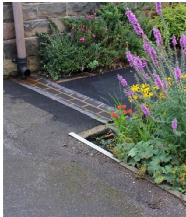
A retrofit downpipe shoe and brick channel into a raingarden
