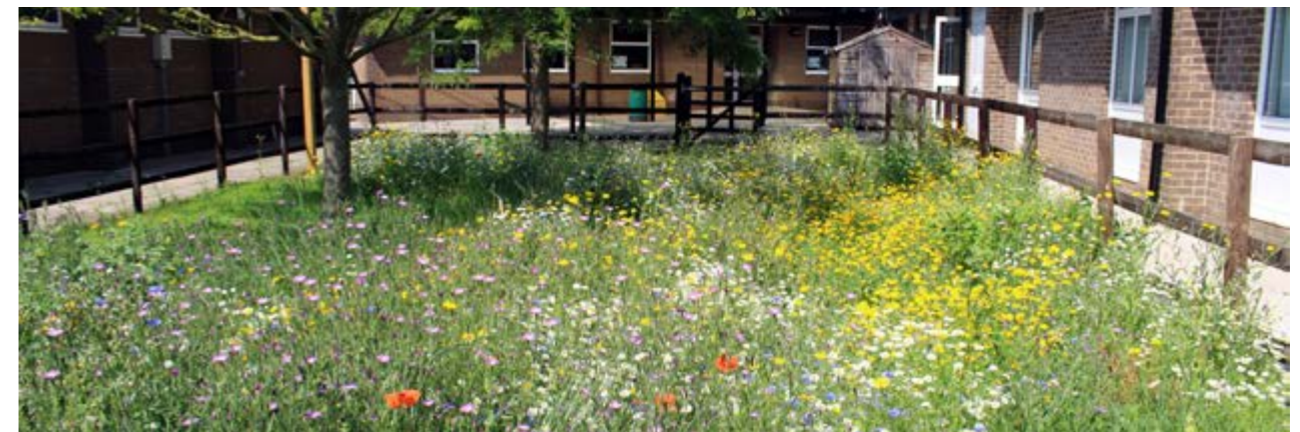
Example of a raingarden managing day-to-day rainfall (e.g. up to the 1 in 10 rainfall event) with flows passing onto subsequent features.
