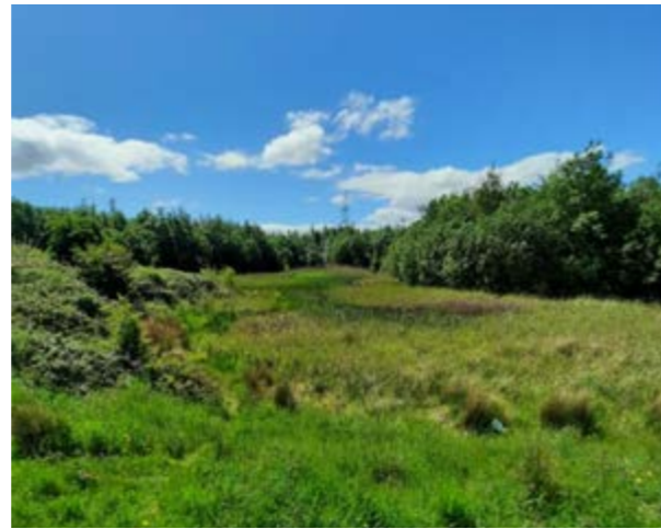
Image: Adamstown Avenue Attenuation Ponds and Wetlands (Constructed c. 2005/6)
