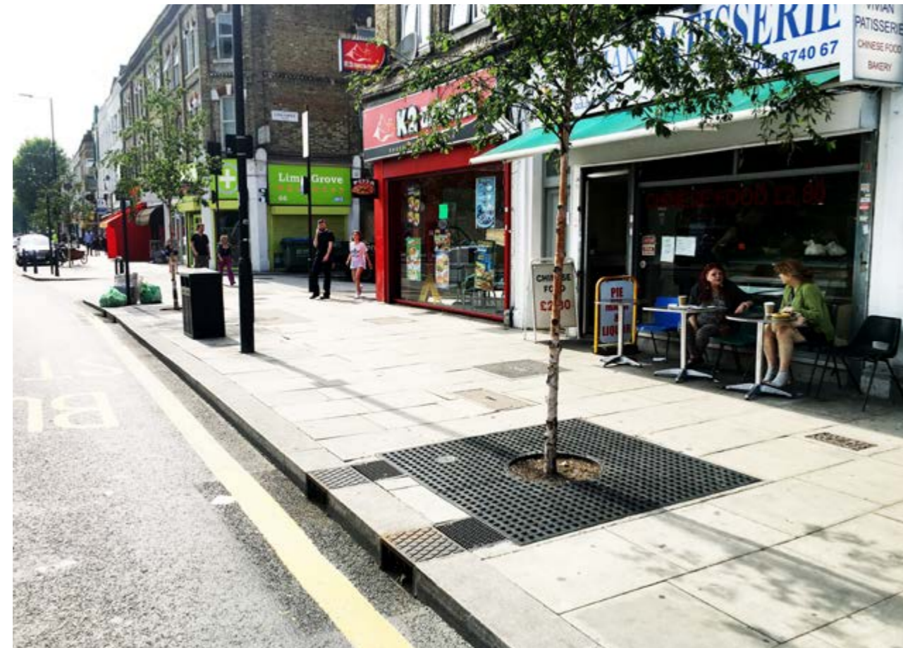
SuDS tree pits managing runoff conveyed through kerb inlets. These two trees share a connected structural soil zone beneath the surface.
