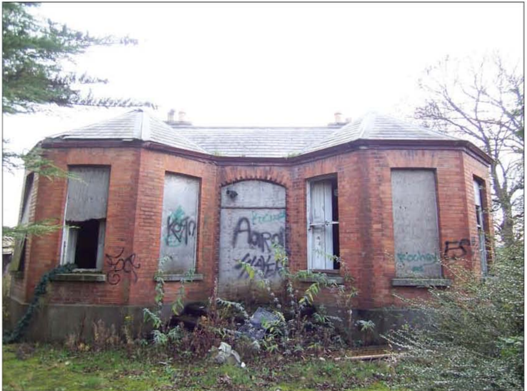
Plate 2 View of Newlands Villa (ID 2) from roadside, facing southeast
