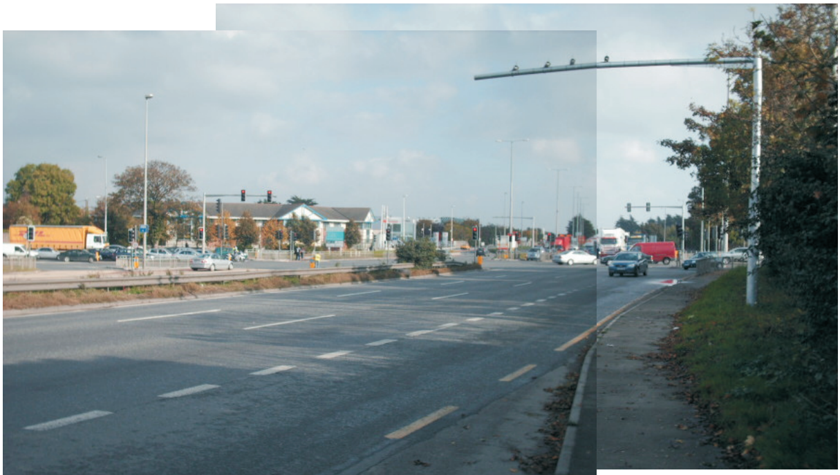
View looking east along the N7 roadway towards the junction Plate 3.1
