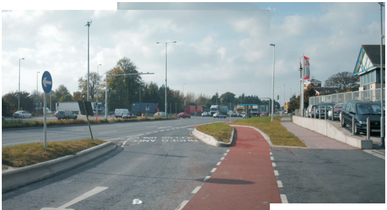
View looking west along the N7 roadway towards the junction Plate 3.2
