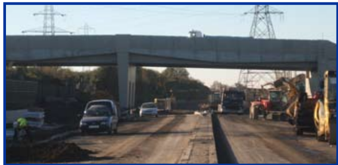
Adamstown Link Road Railway Bridge
