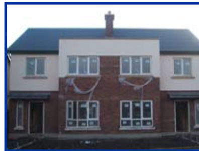
Views of The Paddocks, currently under construction
