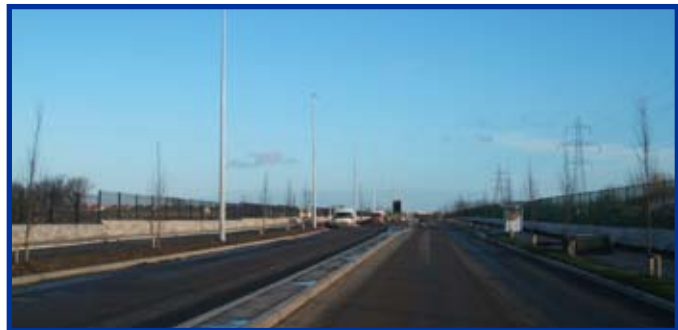
View along Adamstown Link Road, looking east
