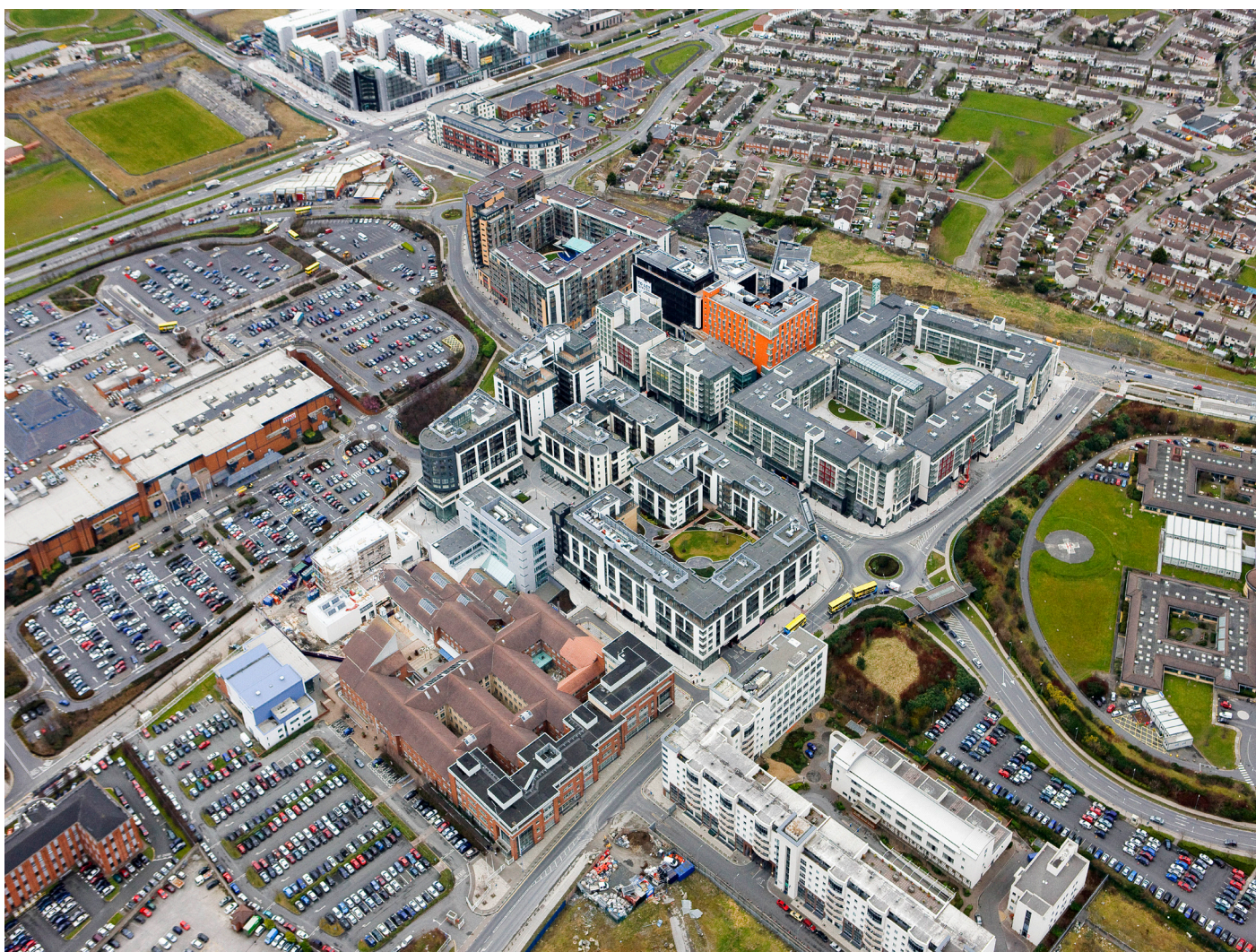
Tallaght Town Centre Aerial Photo 2008
