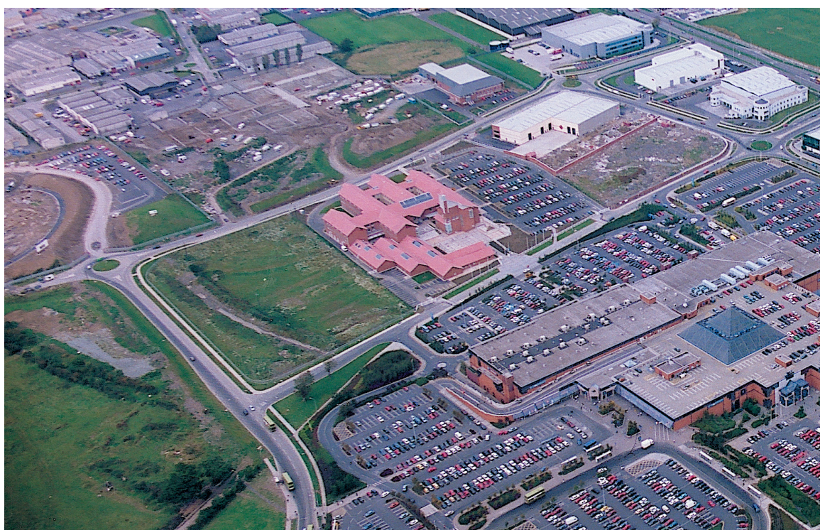
Tallaght Town Centre Aerial Photo 1996
