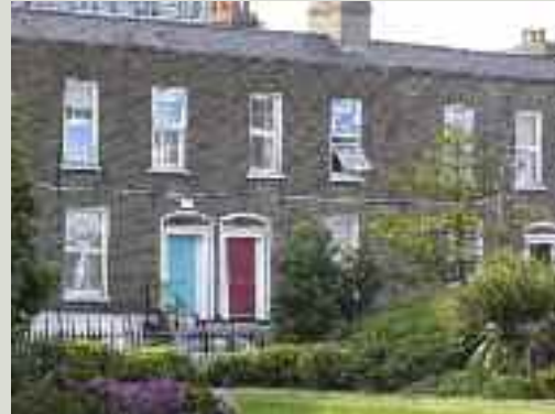
Terraced houses with replacement uPVC-framed windows. These windows are unsympathetic to the character of the houses; opening outward instead of sliding up and down, they disrupt the streetscape; the modern glass creates jarring reflections; while the thick frames contrast poorly with the elegant timber sections of the original sash windows
