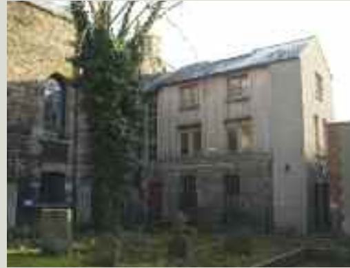
This new extension to the rear of the church provides necessary office accommodation and comprises two storeys built on top of the ruins of the original vestry
