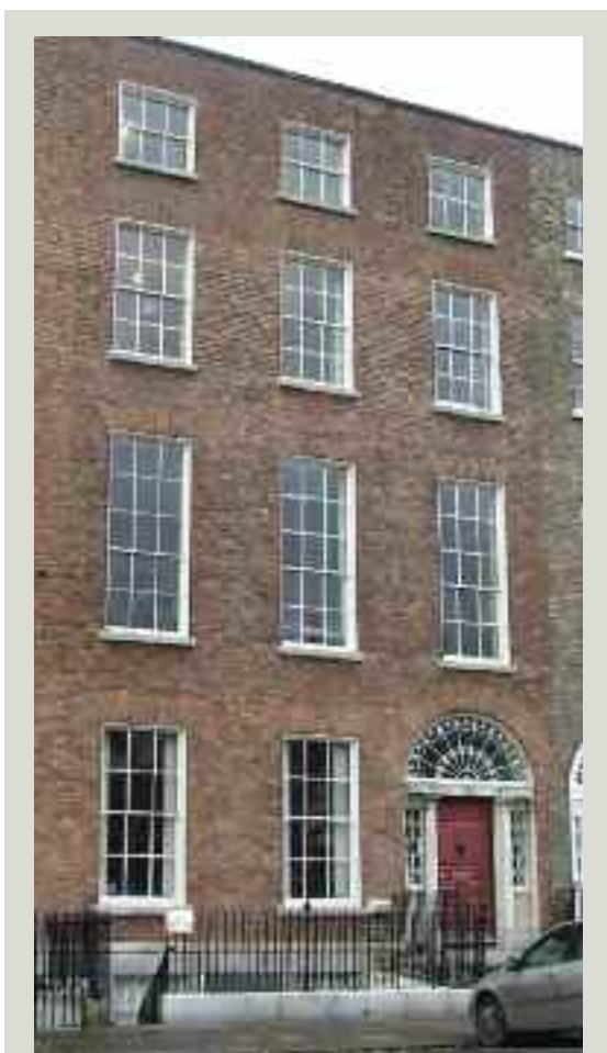
A well-maintained Georgian house with its original timber-framed sash windows
