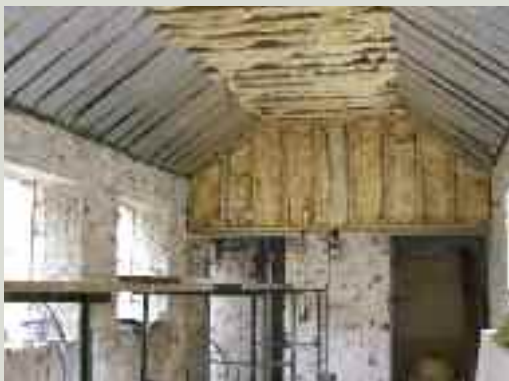
As part of the complete refurbishment of this building, the opportunity was taken to insulate the roof. Rigid insulation has been fitted between the rafters in the sloping sides with quilted insulation fitted between the ceiling joists across the top
