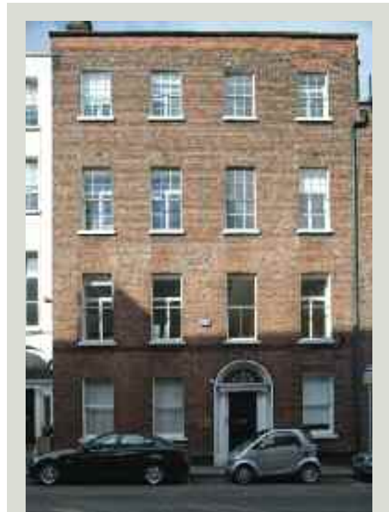
Inappropriate timber-framed secondary glazing with frame proportions that do not match those of the original window, creating a discordant appearance
