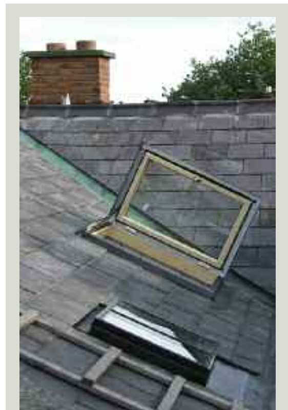
This modern double-glazed skylight allows access to a concealed valley gutter for maintenance inspections and cannot be seen from ground level. It also lets additional natural light into the attic space below
