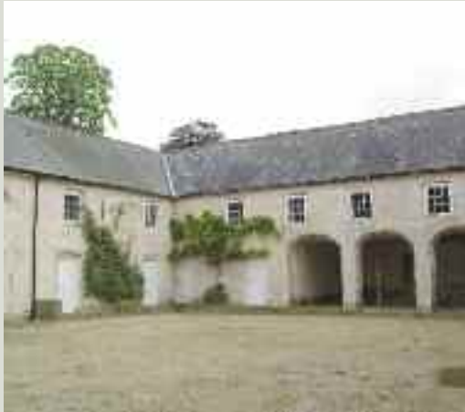
Traditional farm complexes were arranged so that the buildings provided shelter, not only to each other, but also to the outdoor working areas
