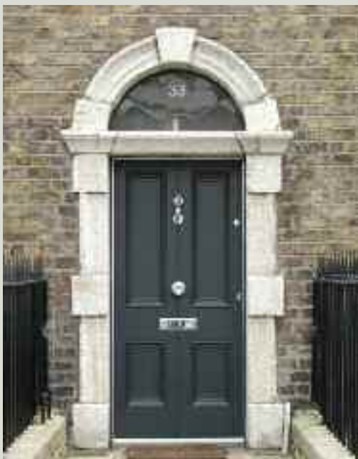
Aluminium draught strips can be seen to all sides of this door. The metal part of these strips, unfortunately visible, can be painted (although it is difficult to achieve successfully) but it is important that the flexible sealant strip is not
