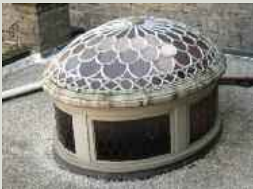
Historic skylights and lanterns, such as this fine example, should be well-maintained but are rarely suitable for thermal upgrading
