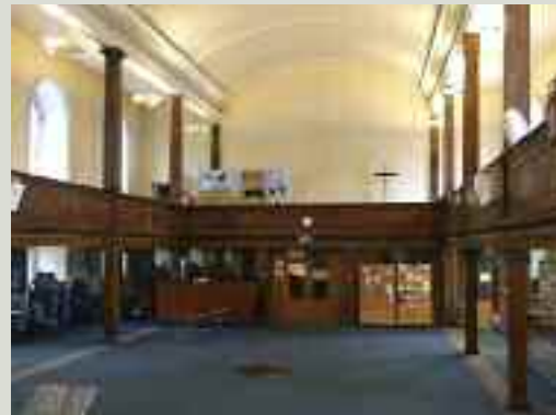
A timber glazed porch was provided inside the main west door, primarily for draught-proofing purposes but also to avoid having to re-hang the external doors, which would otherwise be required to open outwards for emergency egress
