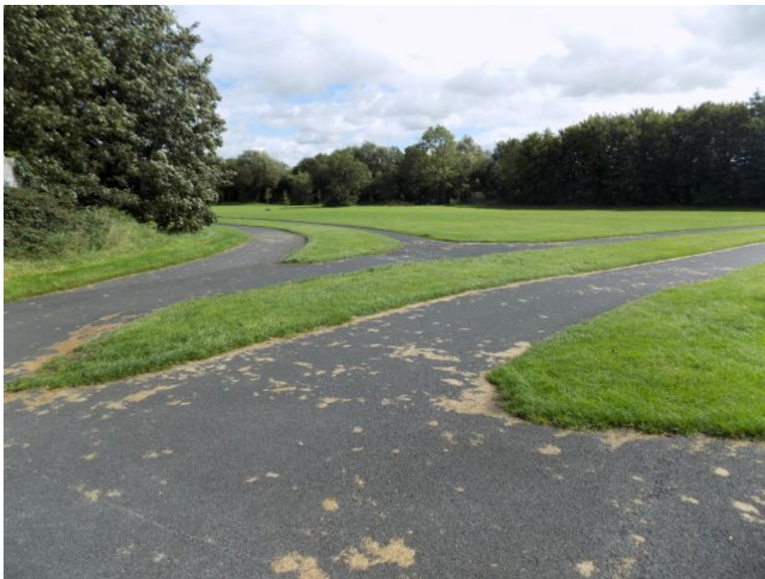
Plate 12 View of site from south west corner looking north east
