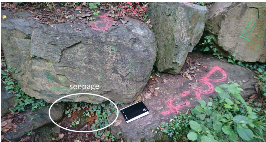
A 7: Seepage D06
