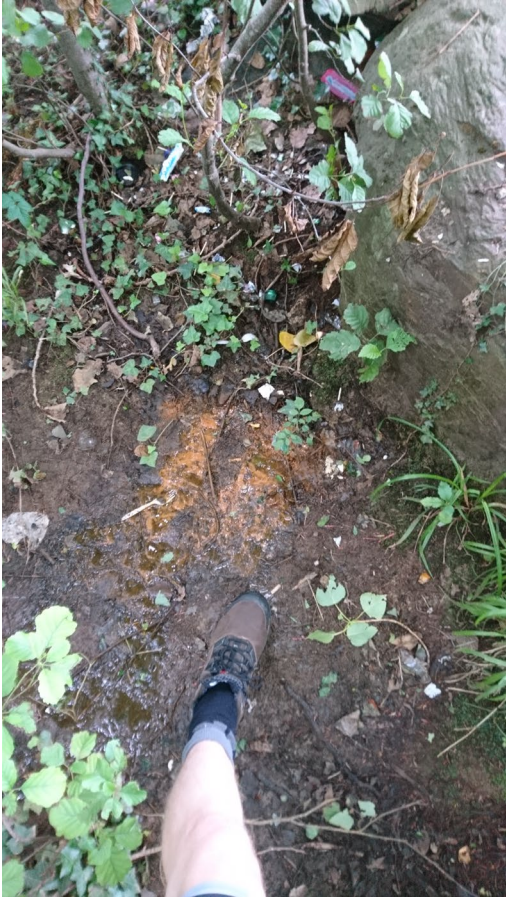
A 3: Seepage D03
