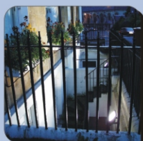
Volume Six Basements
