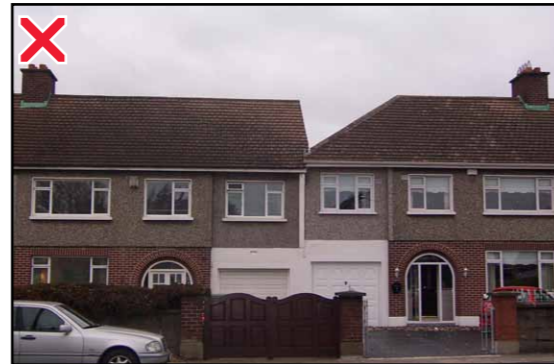
Avoid extending a hipped roof to create a gabled end over a side extension or creating a terraced effect and difficult joins between rooflines
