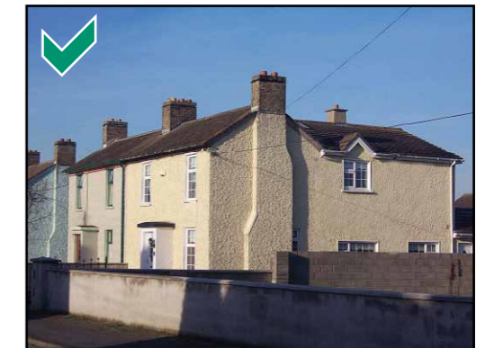
Careful attention to scale and detail is particularly important where large rear extensions are visible from public view
