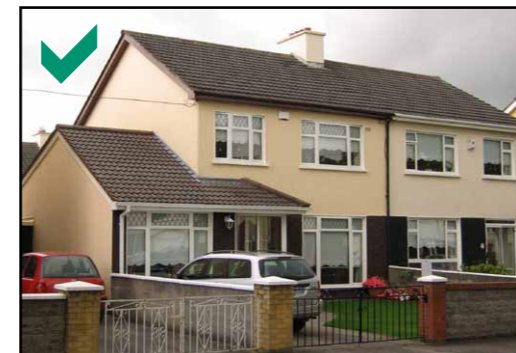
A front extension in keeping with the scale and design of the original house
