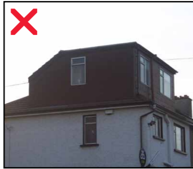
Avoid large and dominant roof extensions and dormer windows that are over-scaled in relation to the roof of the house
