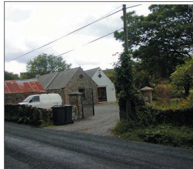
Refurbished Cottage within Study Area
