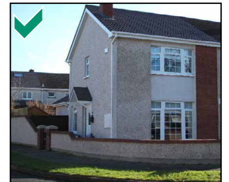
A good example of 'turning the corner'; a side extension on a corner plot that avoids creating blank elevations
