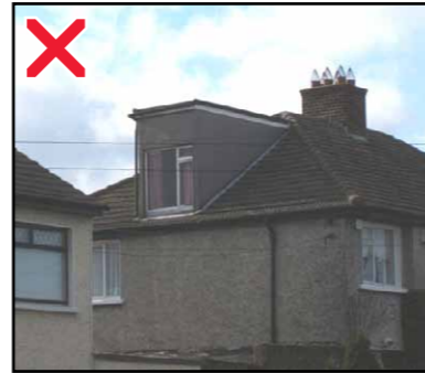
Avoid large and dominant roof extensions and dormer windows that are over-scaled in relation to the roof of the house
