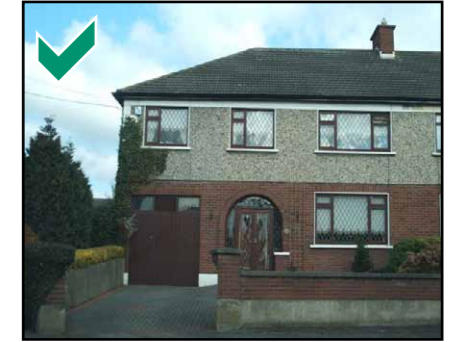
Seamless extension where materials and hipped roof match the original house
