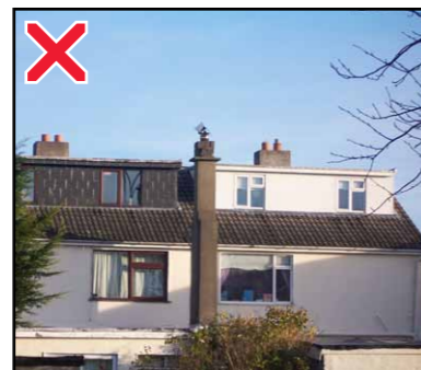
Avoid creating the impression of a 'flat roof' with badly designed roof extensions
