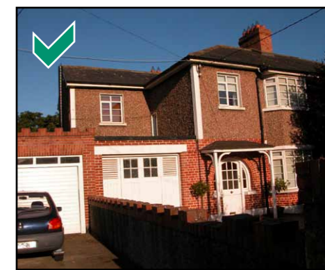
Porches designed to reveal an arched front door and complement the style of the house
