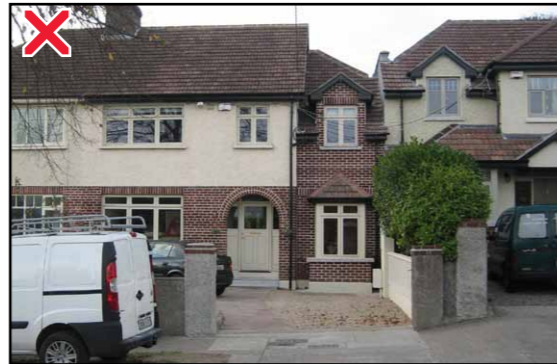
Avoid awkwardly shaped side extensions to houses with hipped roofs as this can result in a visually unbalanced appearance. Note also parapet wall between extensions
