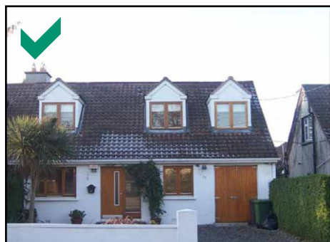
Dormer windows should be located so they do not obscure the ridge line of the roof, are set well above the eaves line and balance the appearance of the main house in terms of design. They should reflect the character, materials and details of the main house.
