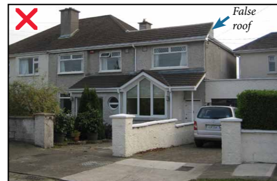
The use of a 'false' roof to the front of an extension is rarely successful
