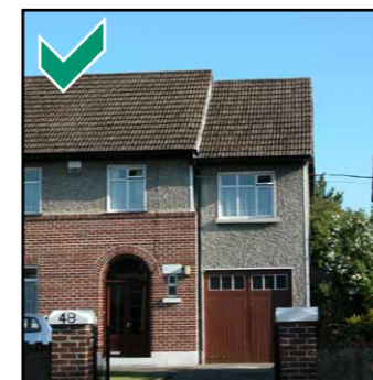
Ancillary extension that is recessed behind the building line
