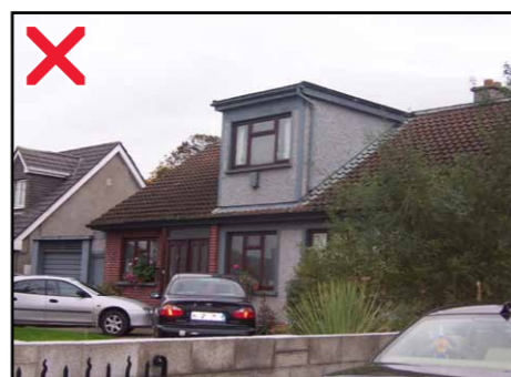
Dormer windows should be located so they do not obscure the ridge line of the roof, are set well above the eaves line and balance the appearance of the main house in terms of design. They should reflect the character, materials and details of the main house.
