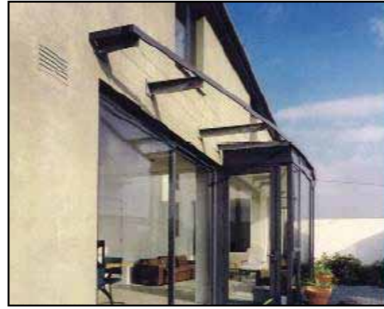
Make the most of south facing elevations with a sunroom or conservatory Source: www.sei.ie
