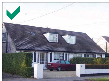
Dormer windows should be located so they do not obscure the ridge line of the roof, are set well above the eaves line and balance the appearance of the main house in terms of design. They should reflect the character, materials and details of the main house.
