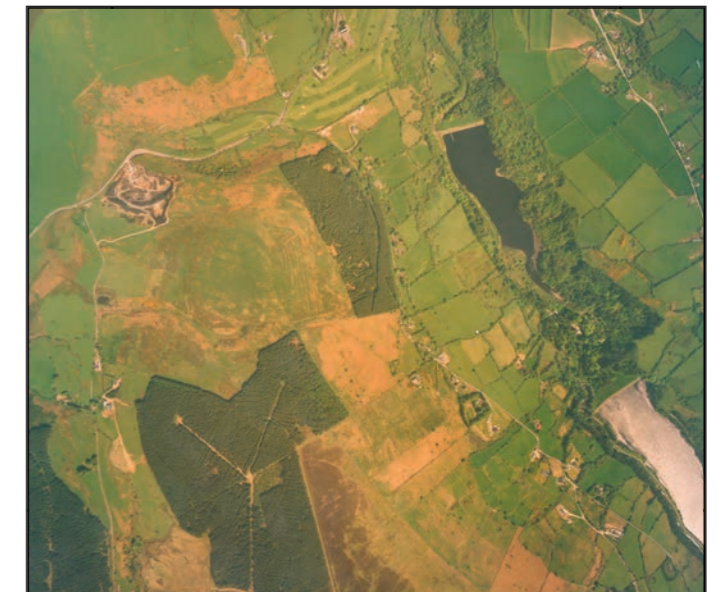
Aerial view of Lower Bohernabreena Reservoir
