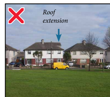
A poorly designed roof extension that does not sit below the ridgelines of the original hipped roof will detract from the appearance and rhythm of hipped roof houses in a visually prominent location
