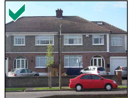
Examples of an 'ancillary' extension that reflects the hipped shape of the original roof
